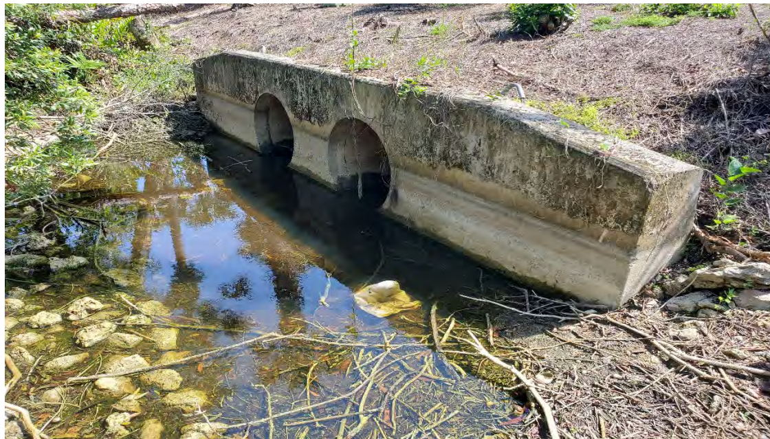
Concrete Headwalls w/ Pipe
