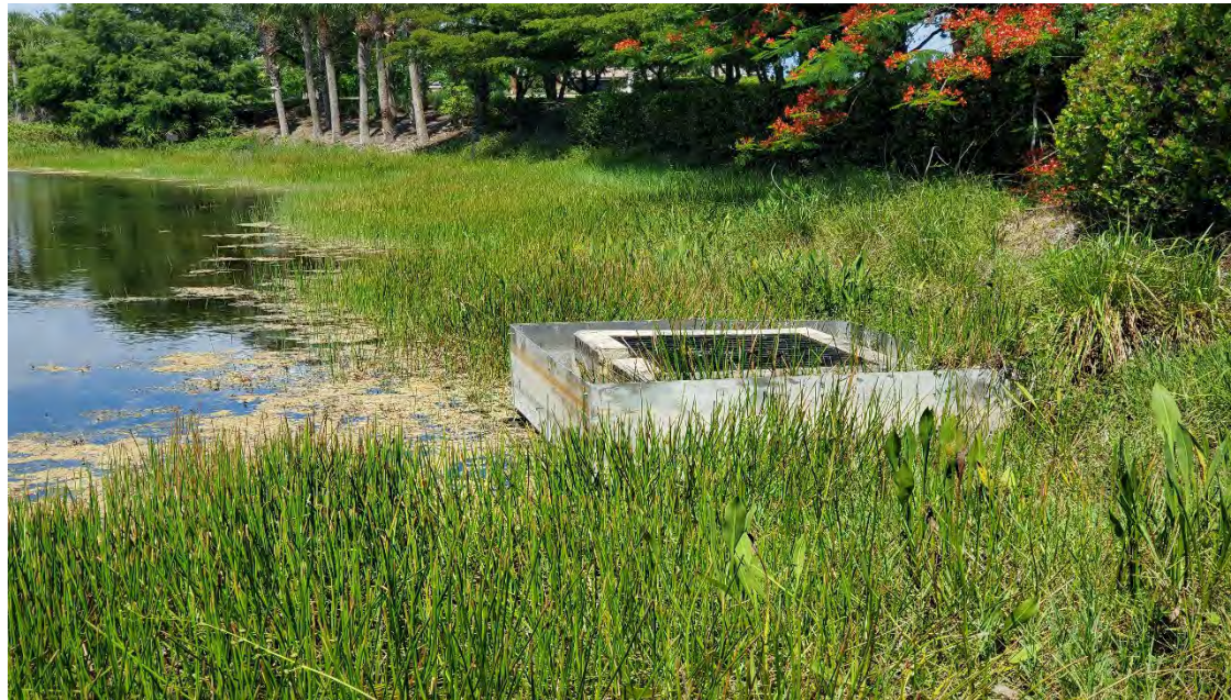
Outfall and Control Structure w/ Drainage Pipe
