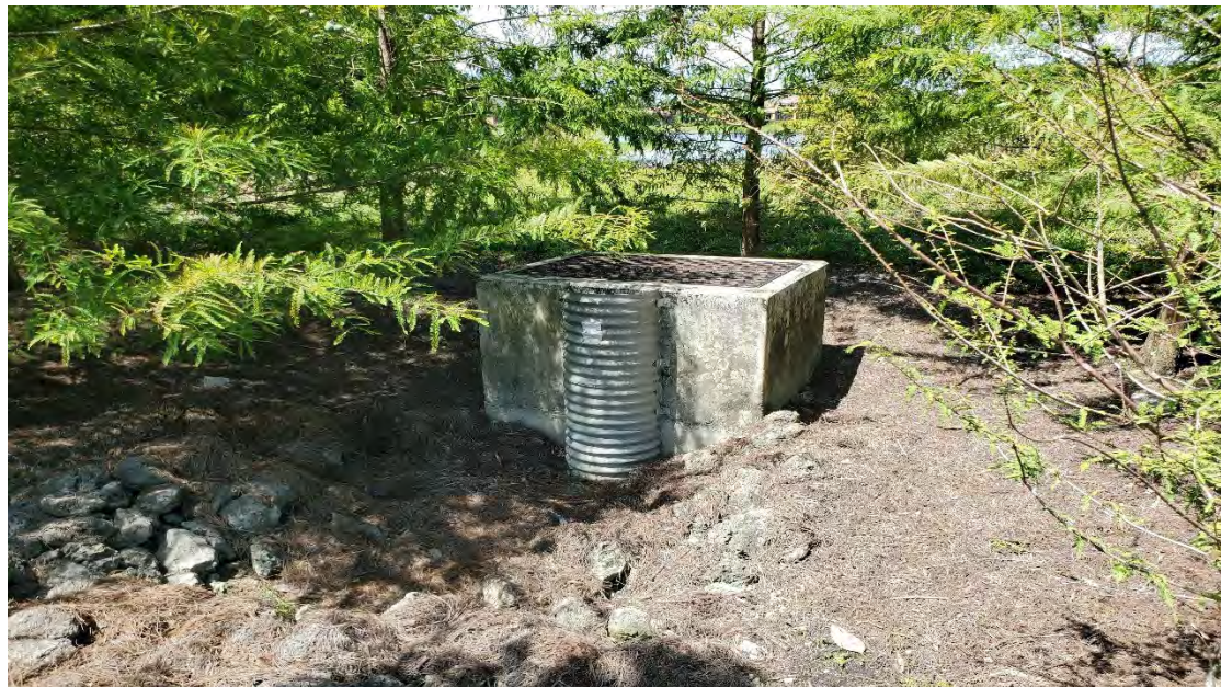
Outfall and Control Structure w/ Drainage Pipe
