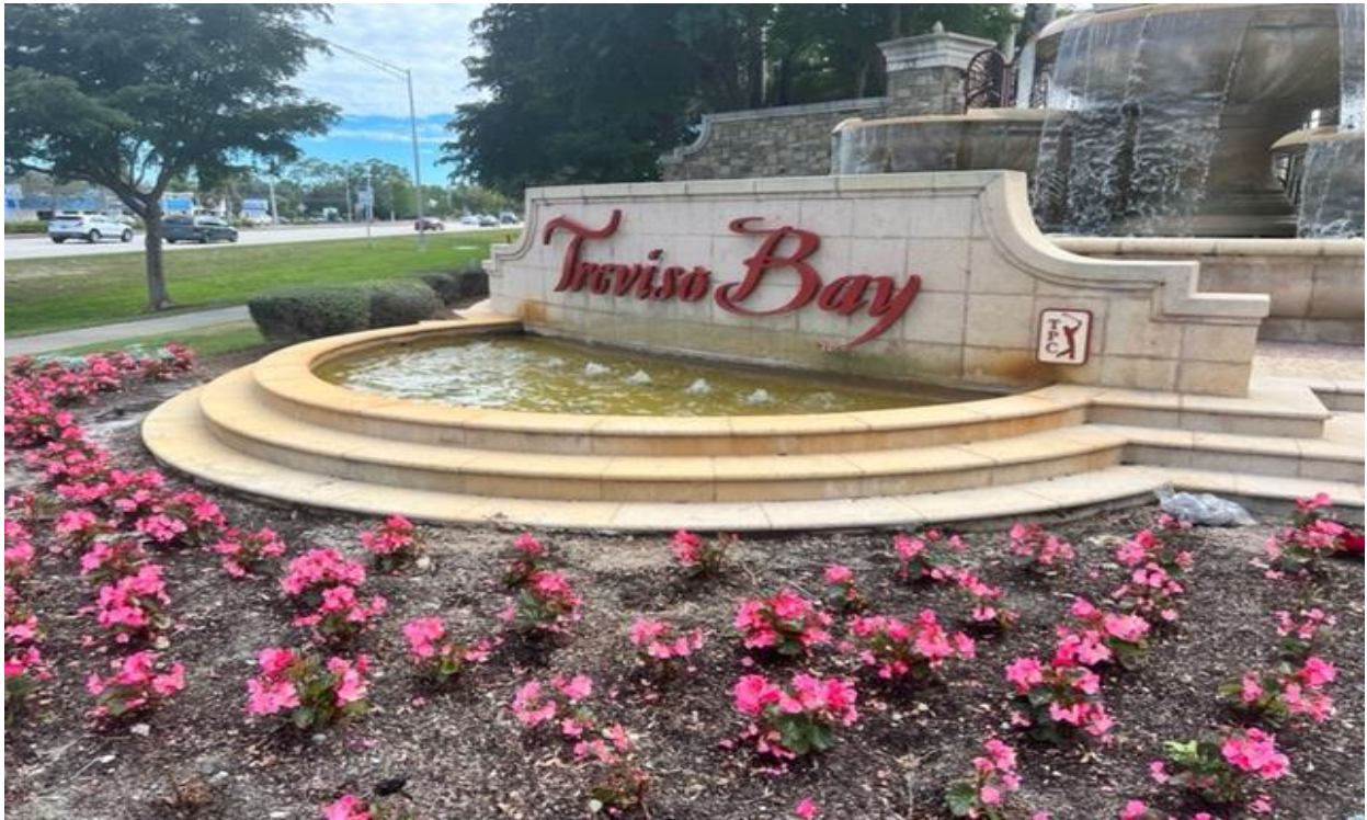
Front Entrance East Fountain That Is Not Working Properly
