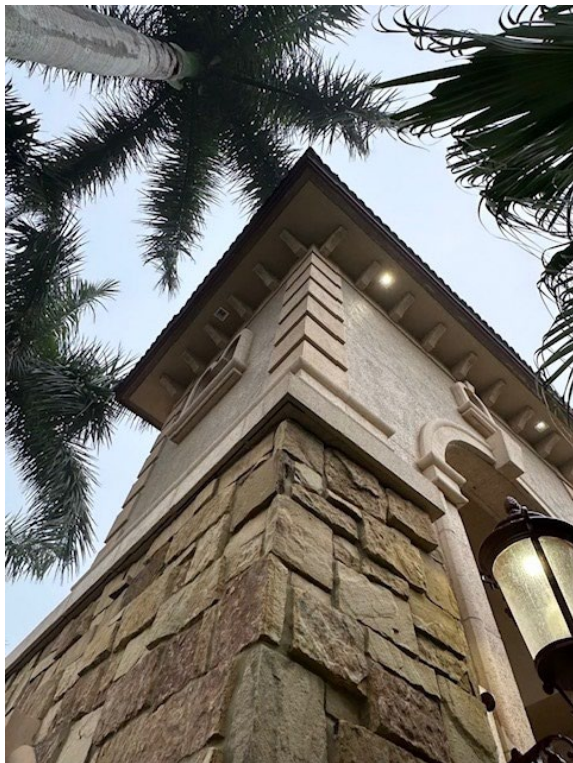
Bridge lighting that was replaced along the front entrance.
