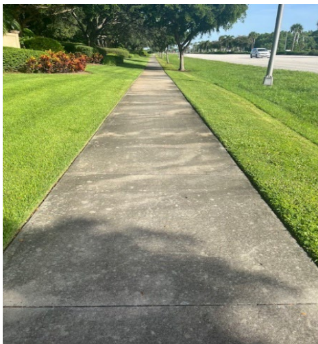
Before Pedestrian sidewalk was pressure cleaned.
