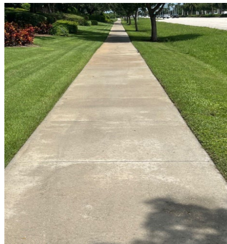
After Pedestrian sidewalk was pressure cleaned.
