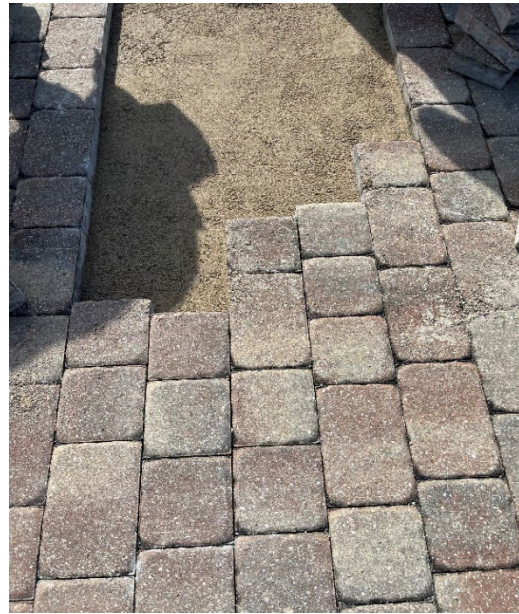
New pavers being installed.
