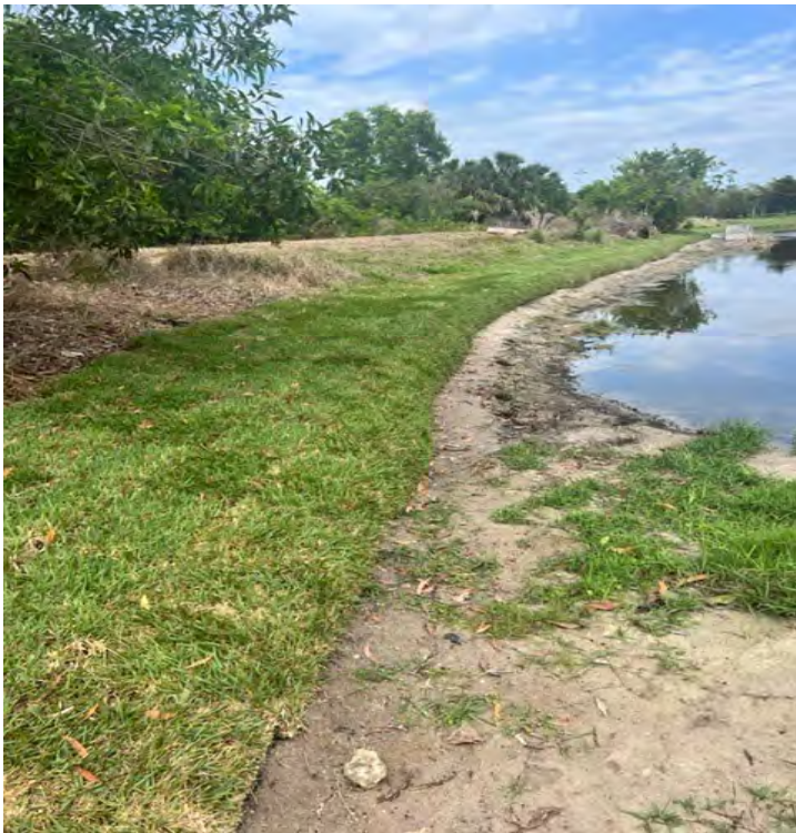
LAKE BANK RESTORATION ON LAKE 21
