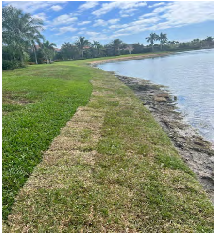
LAKE BANK RESTORATION ON LAKE 21
