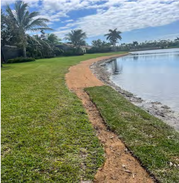
LAKE BANK RESTORATION ON LAKE 21
