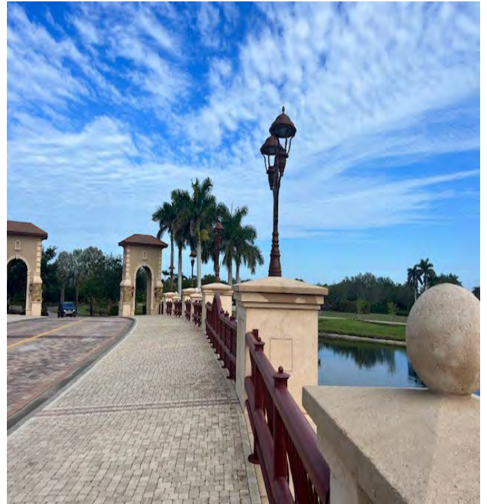
BRIDGE LIGHTING AT FROM ENTRANCE
