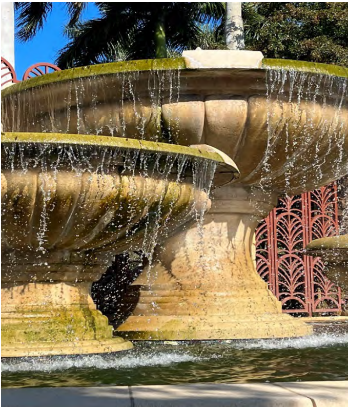
ENTRANCE FOUNTAIN BEFORE PRESSURE WASHING
