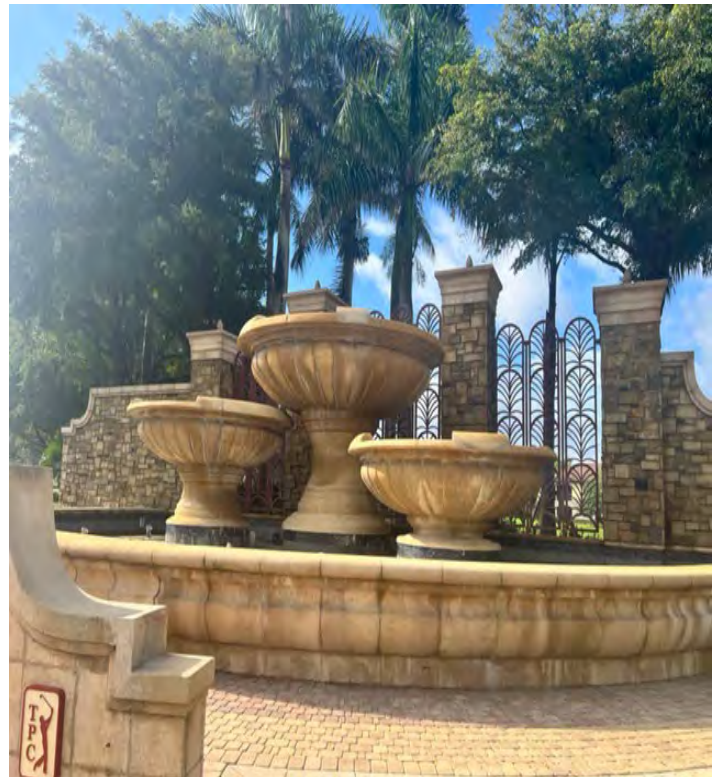
ENTRANCE FOUNTAIN AFTER PRESSURE WASHING
