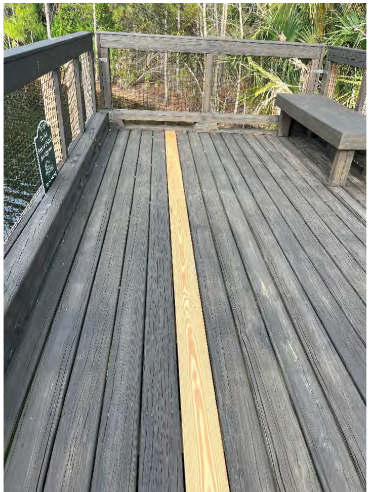
New board installed.
