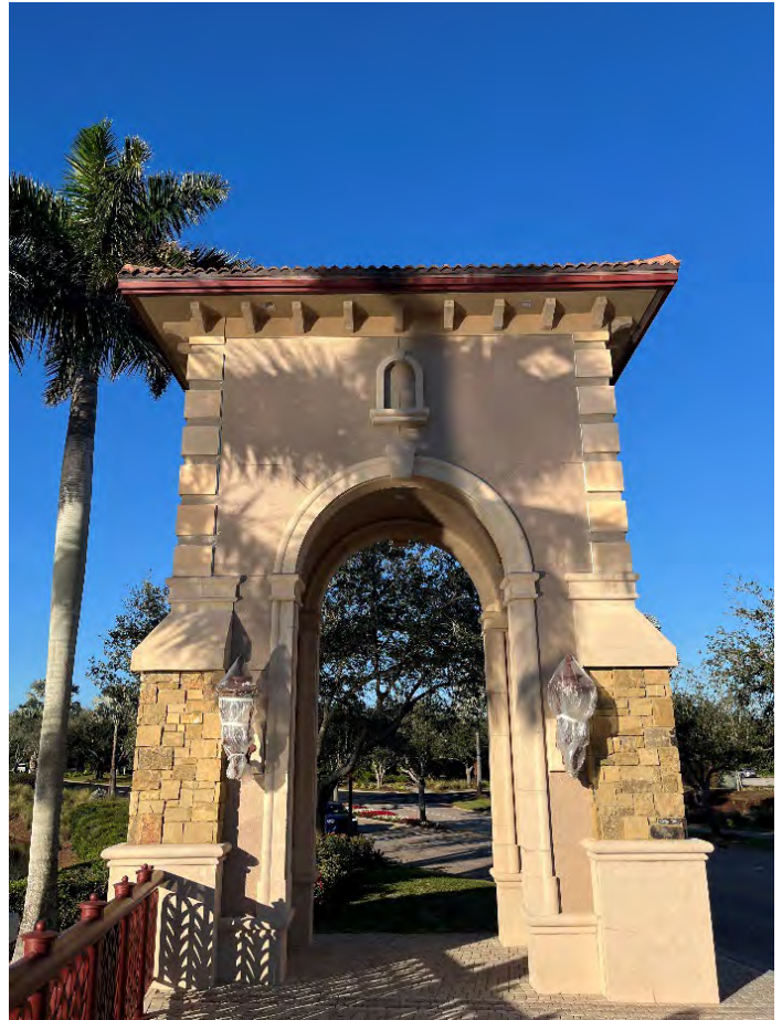
Bridge lights covered during painting.
