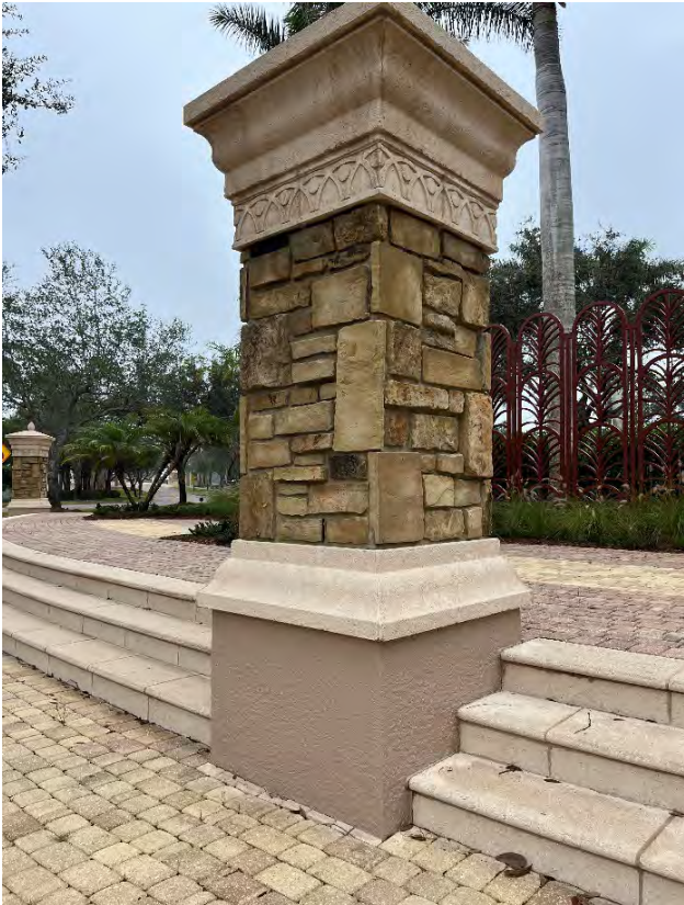
Painting of the main entrance progress.
