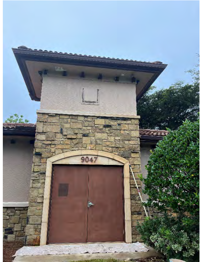
Painting of the main entrance progress.
