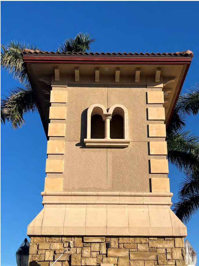
Painting in progress at the entrance.
