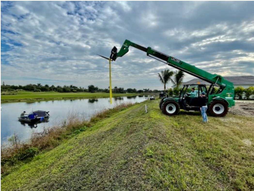
Figure 2. Sonic Buoy and anchor deployment at one of the experimental lakes.
