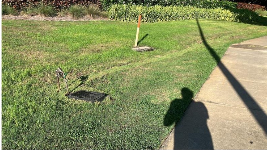
Domestic water service connection and backflow assembly for the east fountain, with turf restored along the trench alignment.
