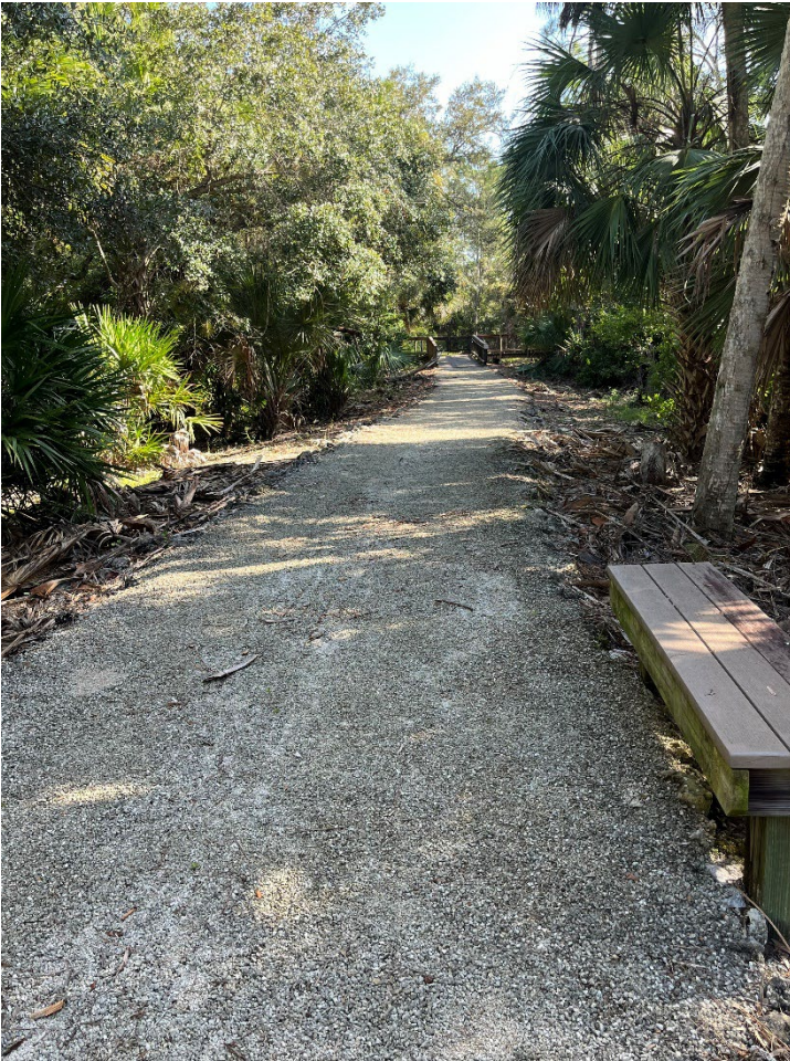
Debris blown off trail.
