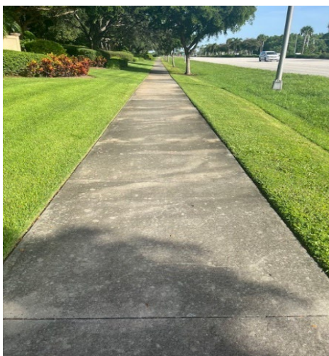
Before Pedestrian sidewalk was pressure cleaned.
