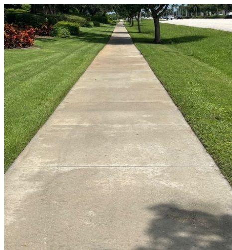
After Pedestrian sidewalk was pressure cleaned.
