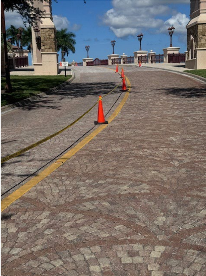
New paver install and sealing
