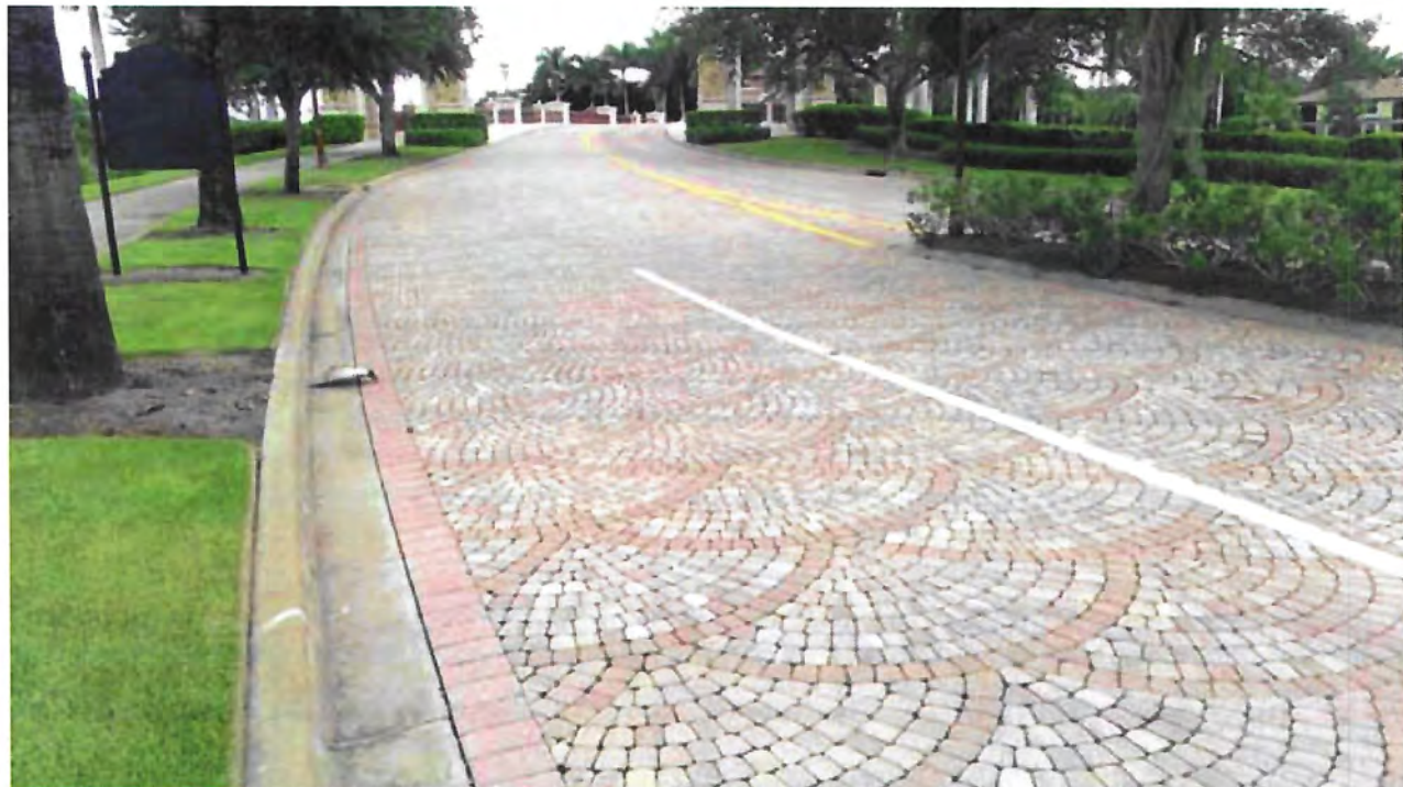
Pavers - Treviso Bay Blvd
