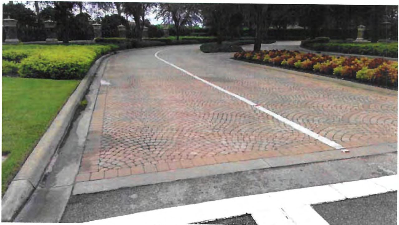
Pavers - Treviso Bay Blvd
