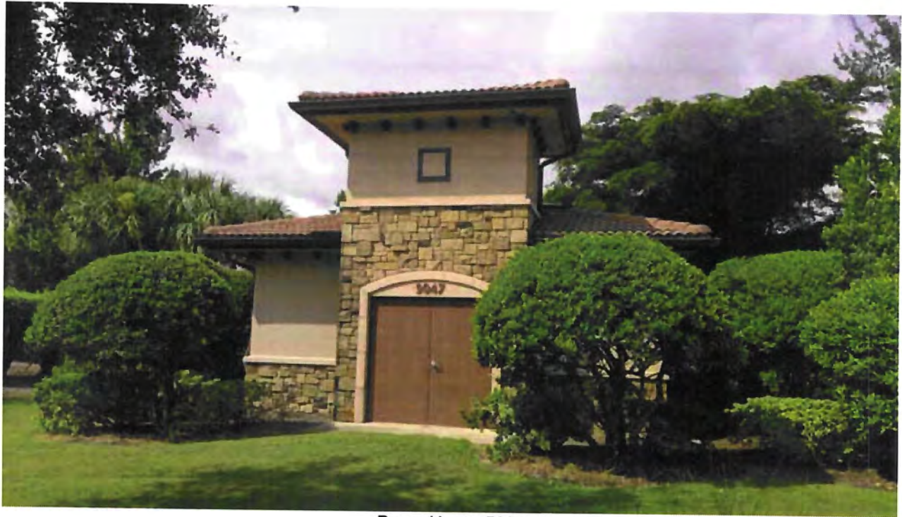
Pump House Bldg
