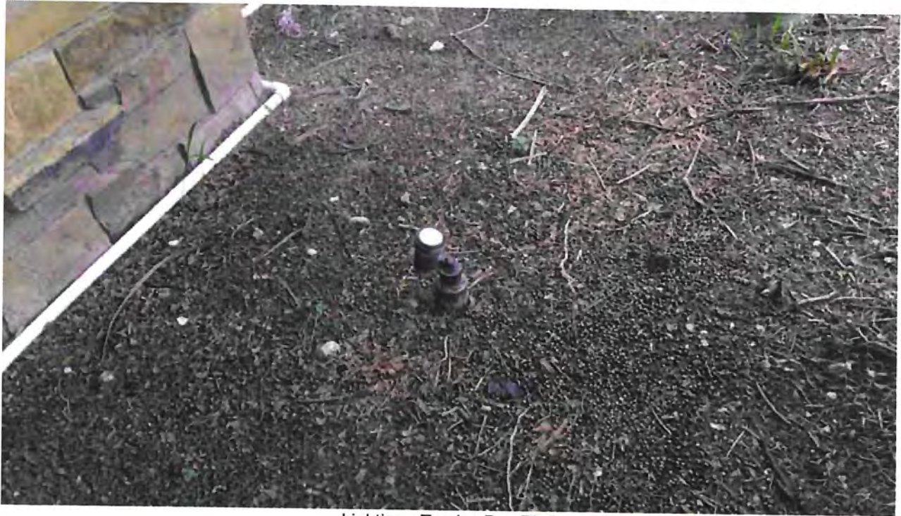
Lighting - Treviso Bay Blvd
