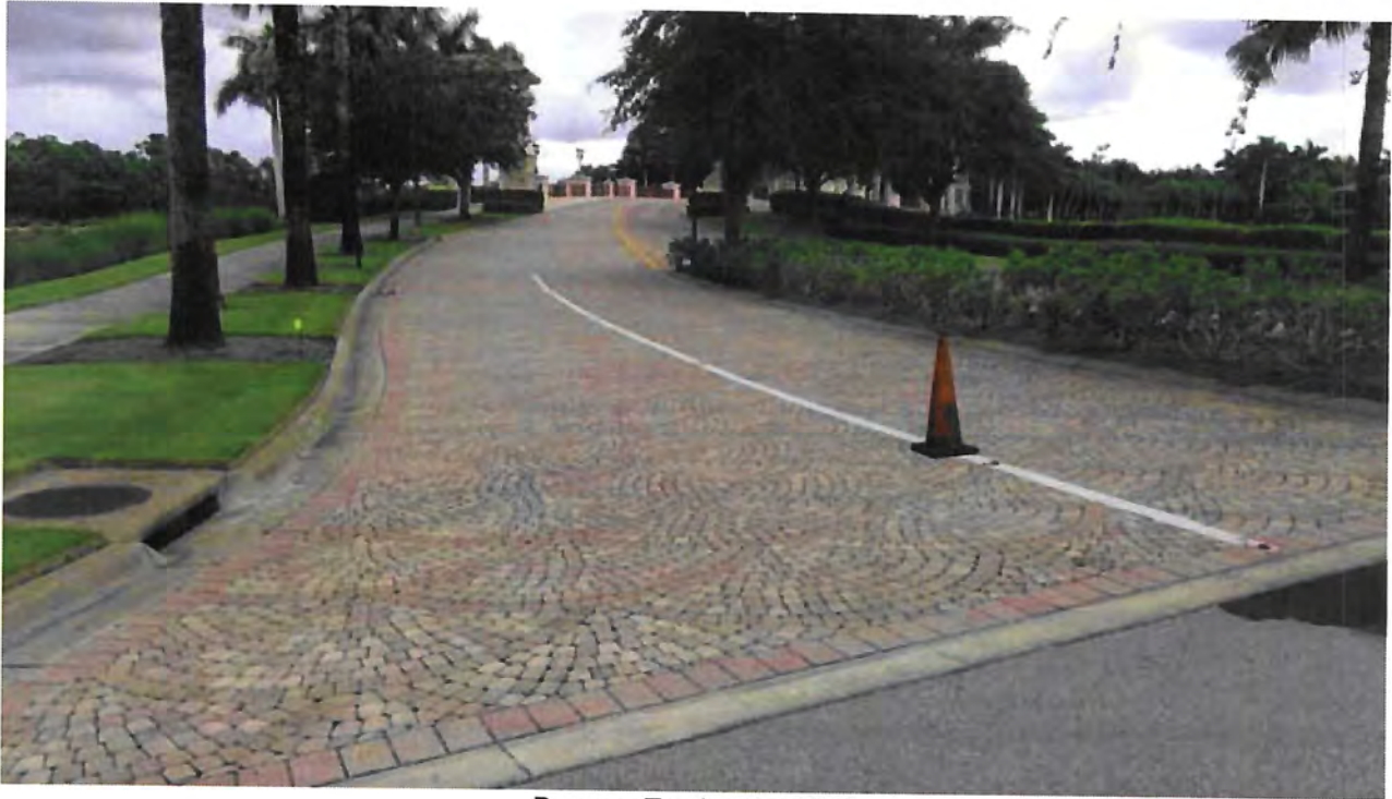
Pavers - Treviso Bay Blvd
