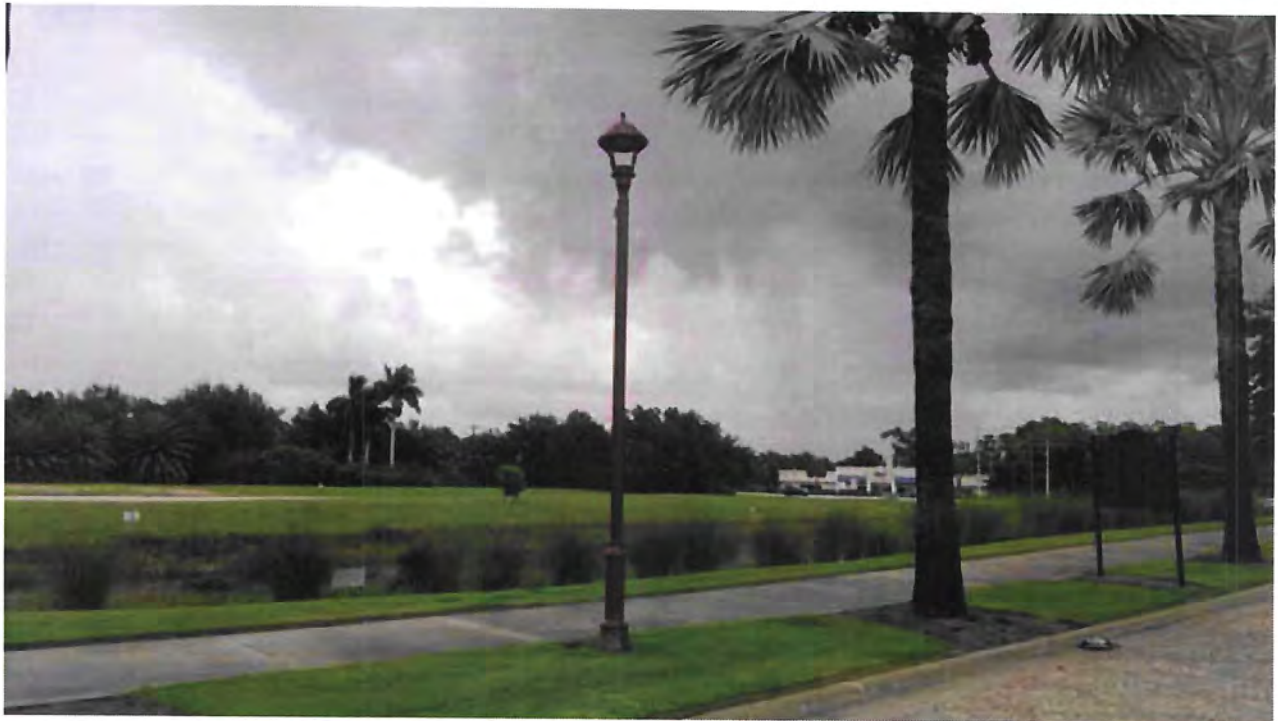
Lighting - Treviso Bay Blvd
