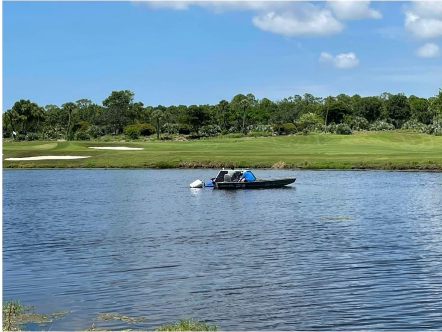
Photos of maintenance work in experimental lakes TB3, TB7 and TB8 on September 8, 2021
