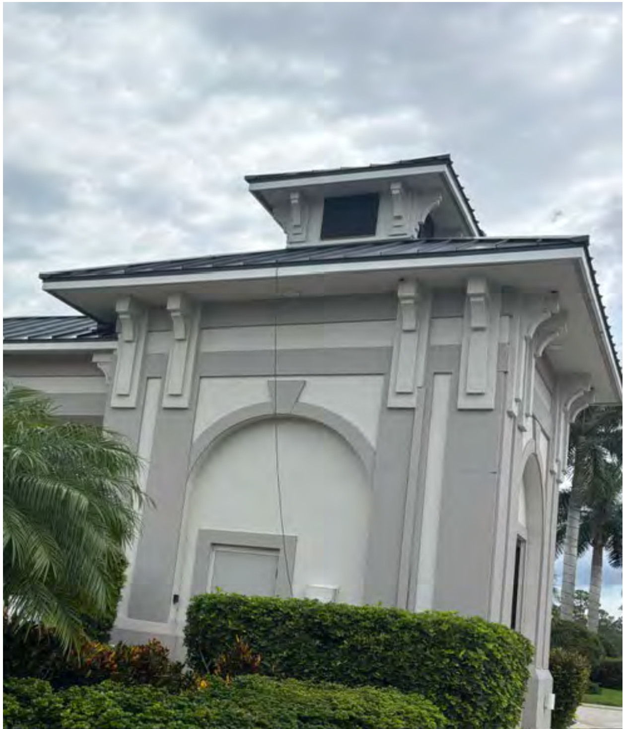
Roof Cable on outside of Guard House
