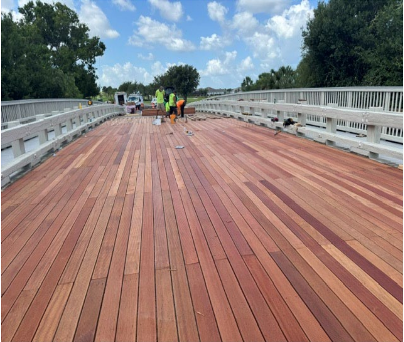
Construction on Bridge No. 2
