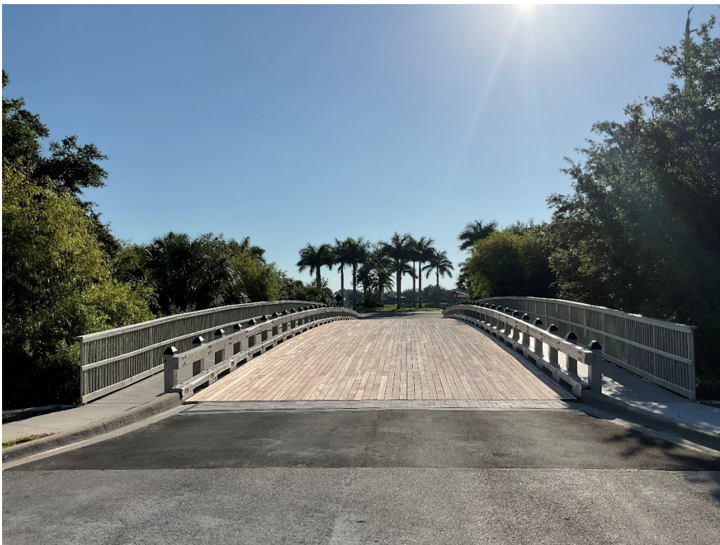
Bridge No. 1 Completed
