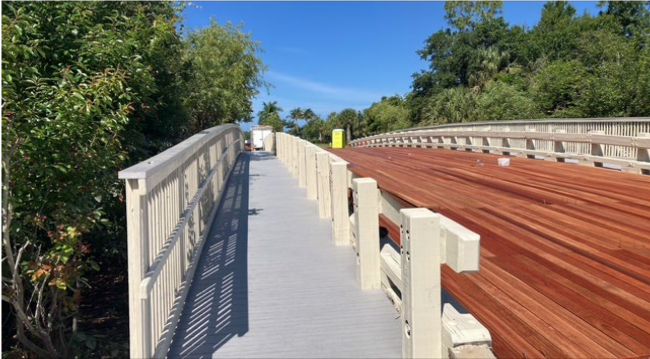
Bridge progress – To be completed by 5/26
