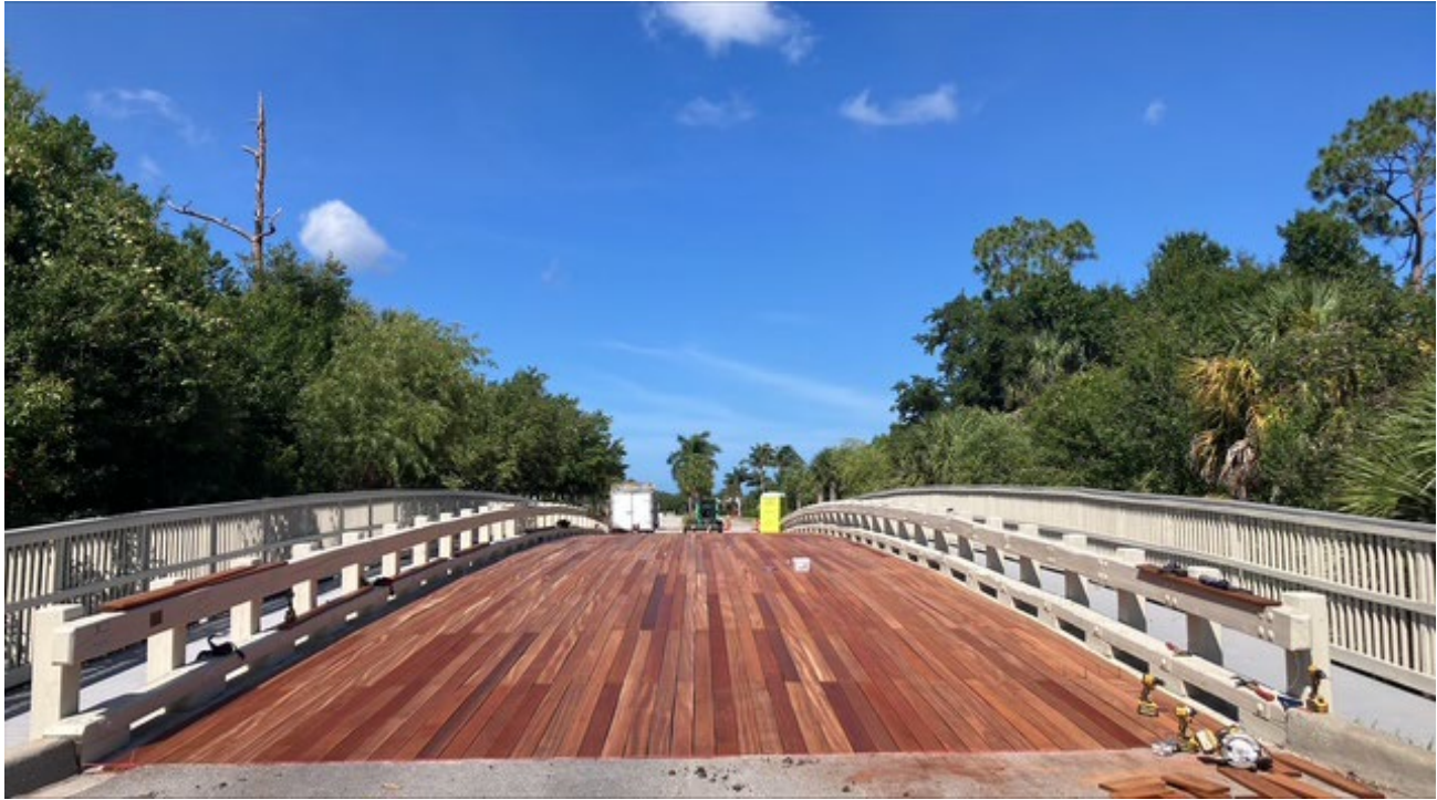
Bridge progress – To be completed by 5/26
