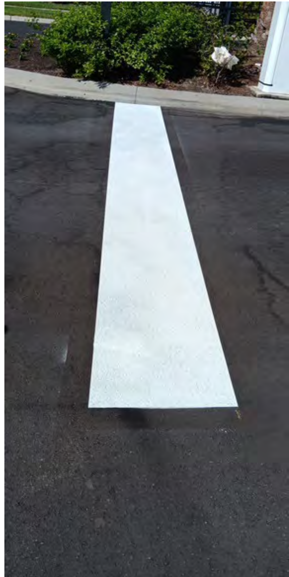
18" Stop Bar Back Entrance
