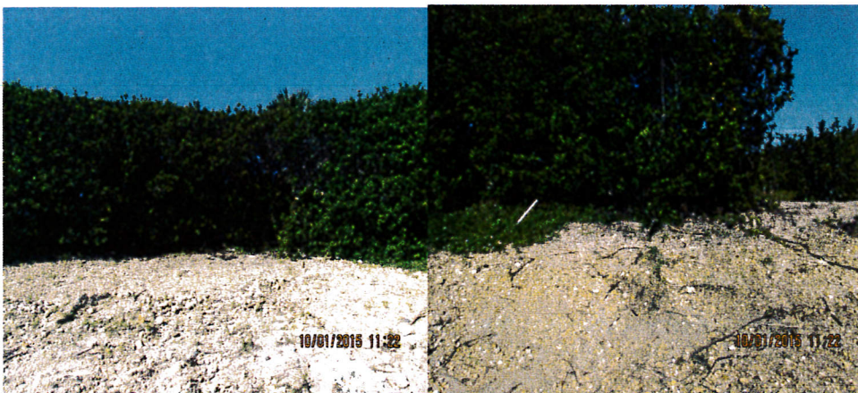
Damaged berm from erosion, awaiting sod installation
