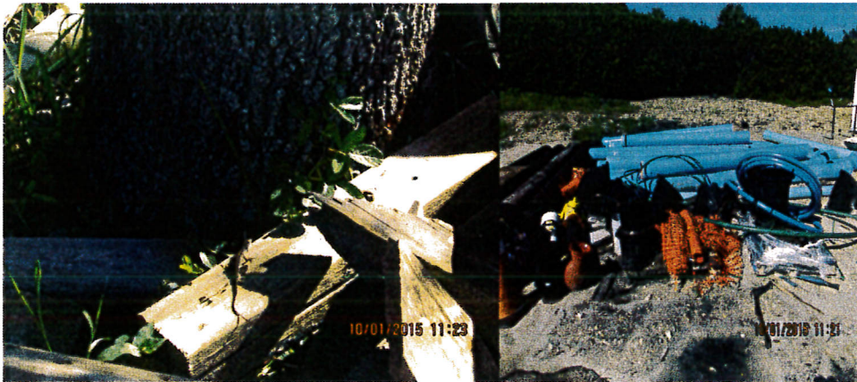
Material storage around tree roots and berm
