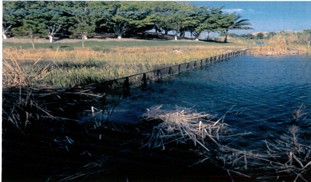
Metal fencing on-top of concrete overflow weir on south side of lake
