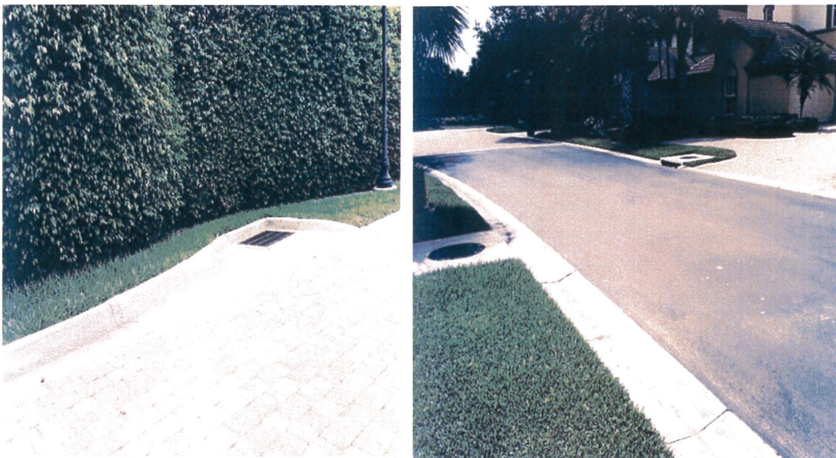
Residential drainage structures for stormwater run-off
