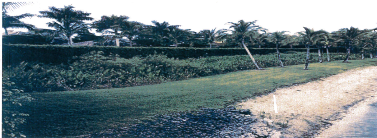
Wet retention area within stormwater system
