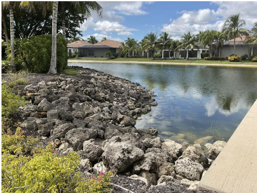
Rip-rap shoreline stabilization along a residential lake bank.
