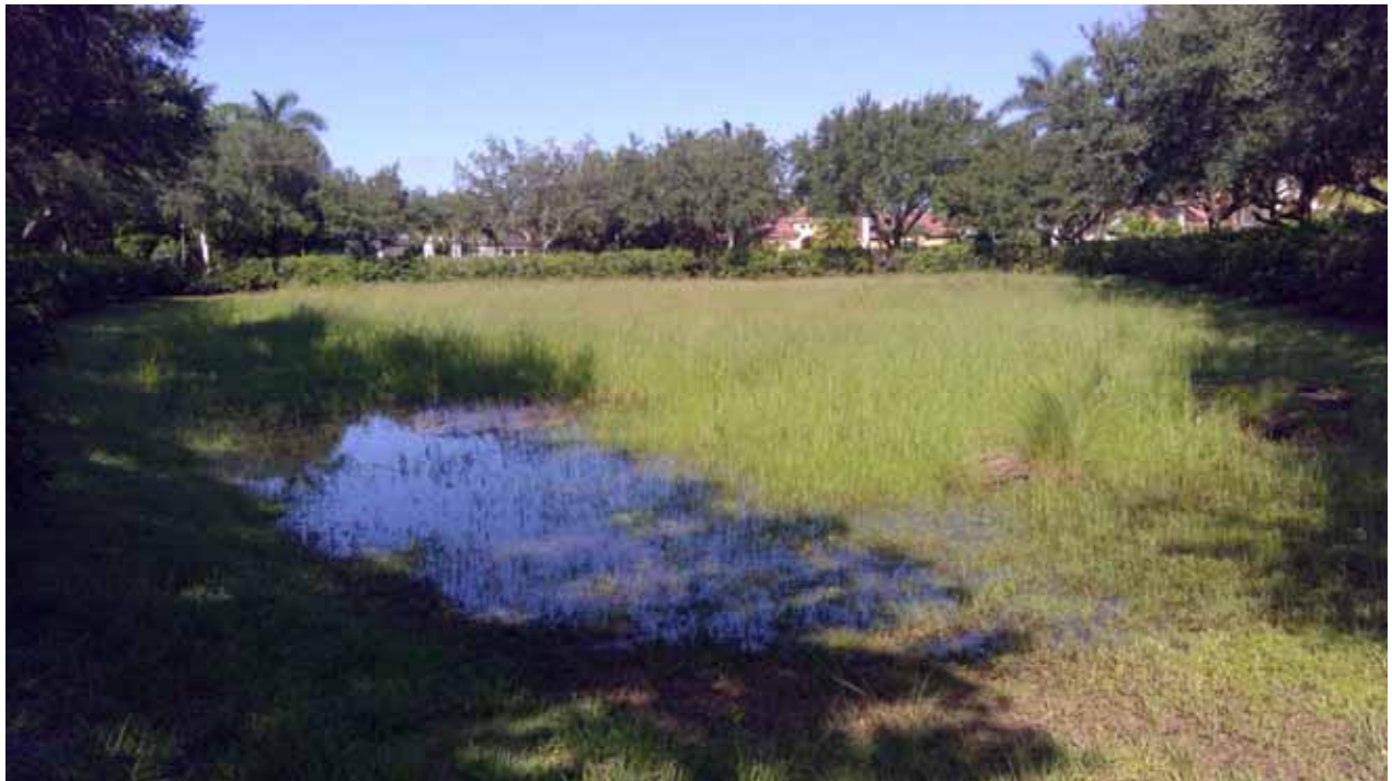
Dry Detention Area #2
