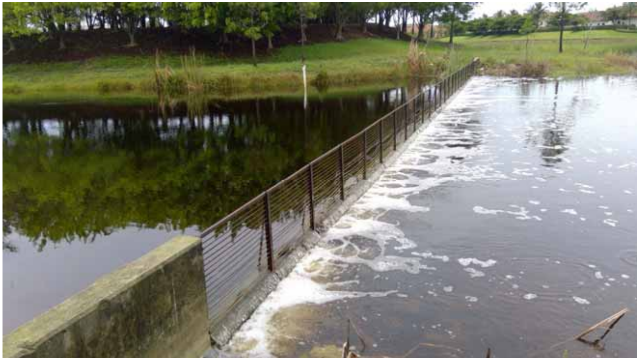
Concrete Weir (FGCU)
