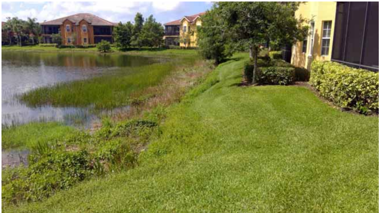
Lake Embankment - 3D
