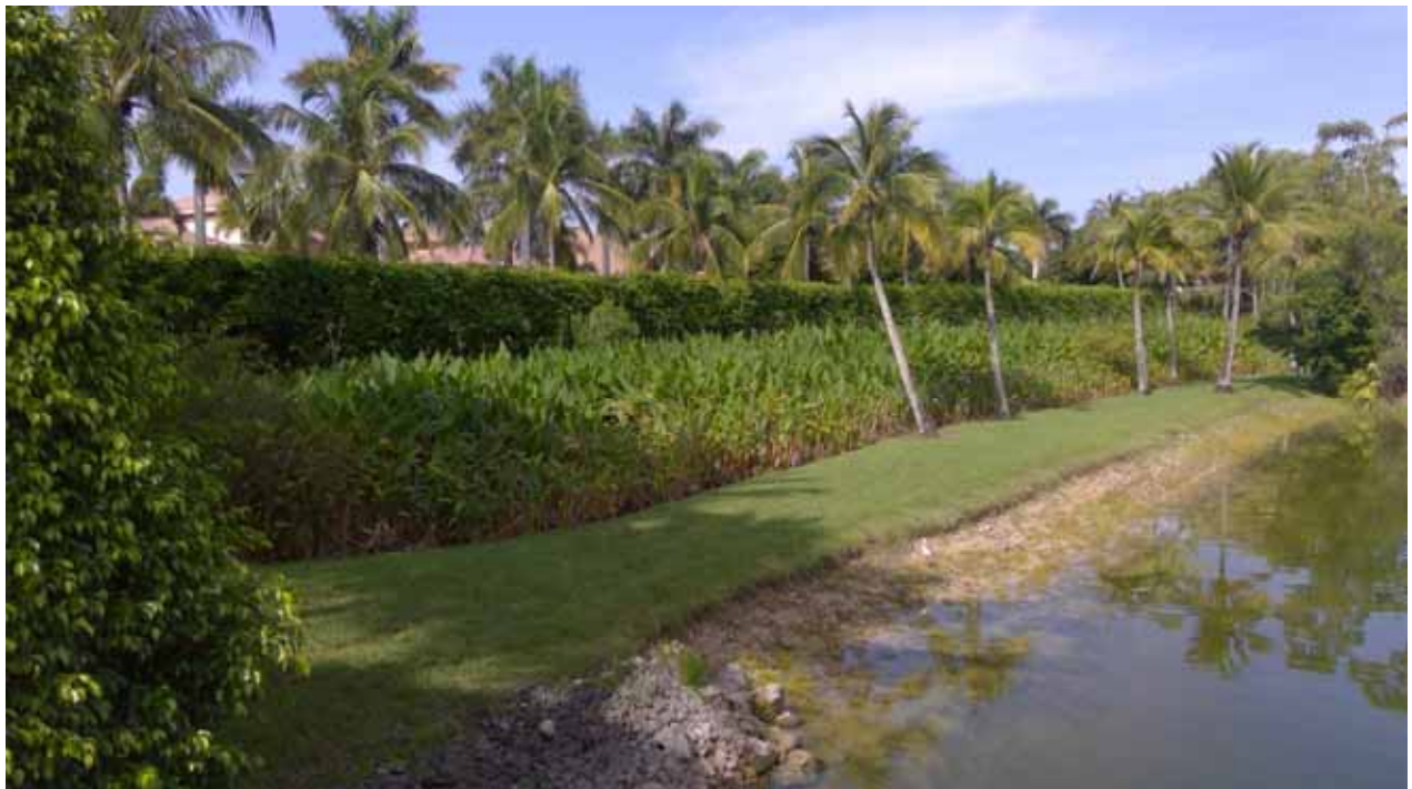
Dry Detention Area #3
