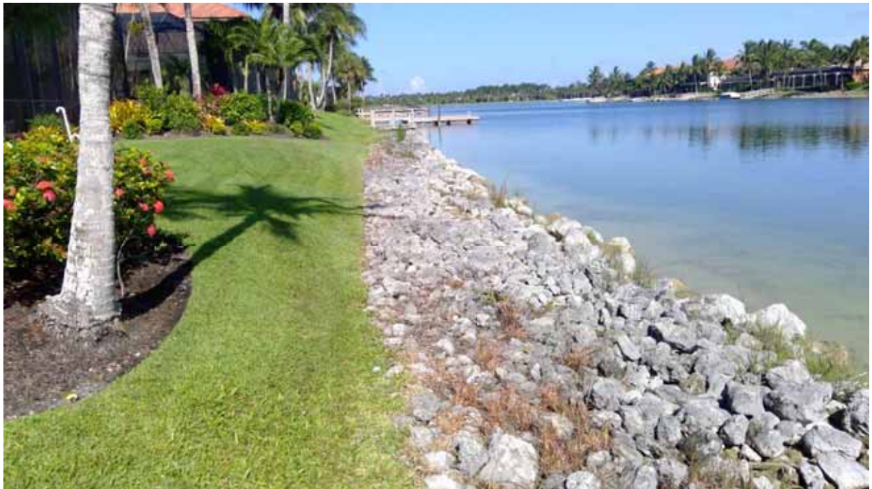
Lake Embankment - 5/6 South
