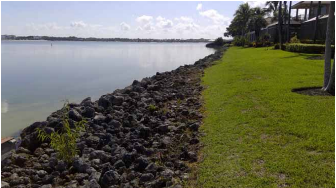
Lake Embankment - 5/6 South
