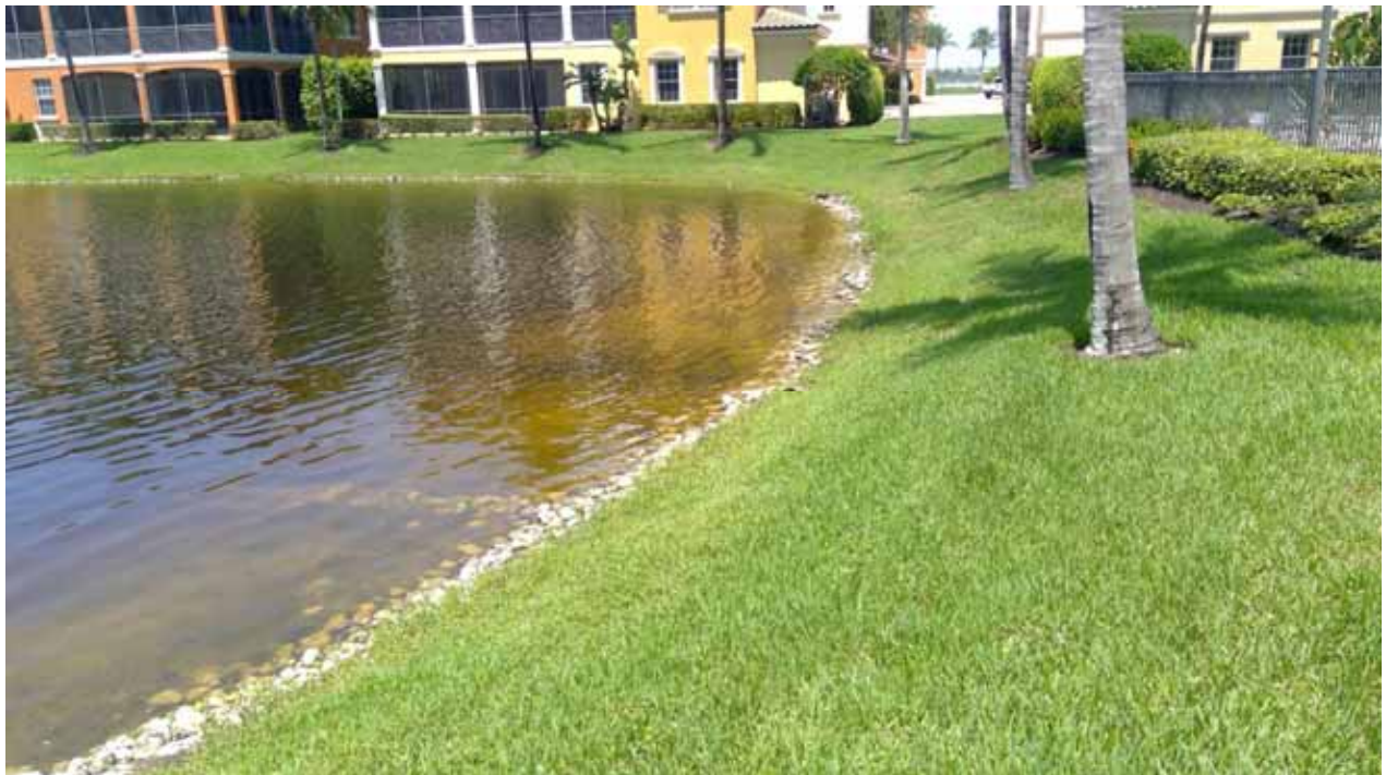
Lake Embankment - Via Milano Dr
