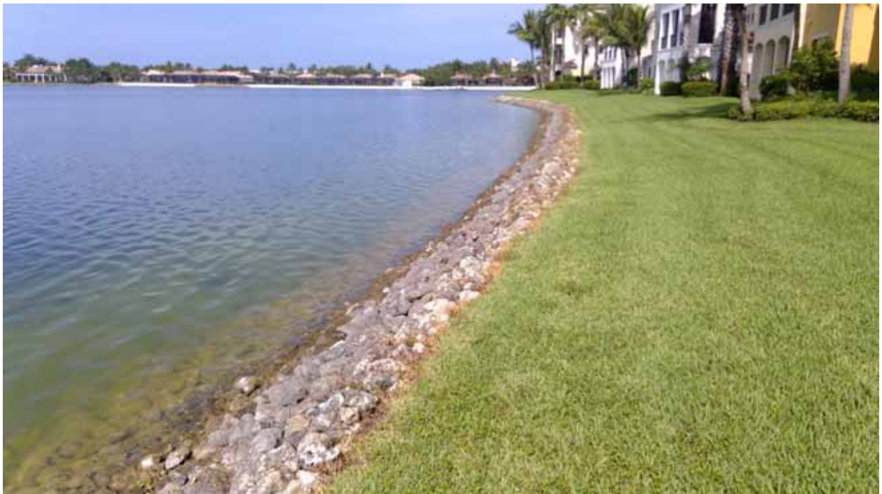
Lake Embankment - 5/6 South
