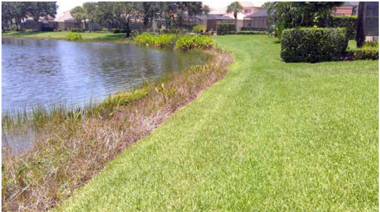
Lake Embankment - 1C
