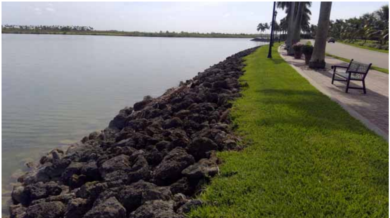
Lake Embankment - 5/6 North
