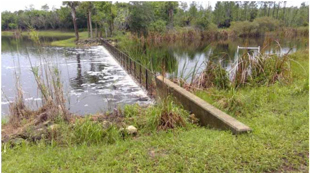
Concrete Weir (FGCU)
