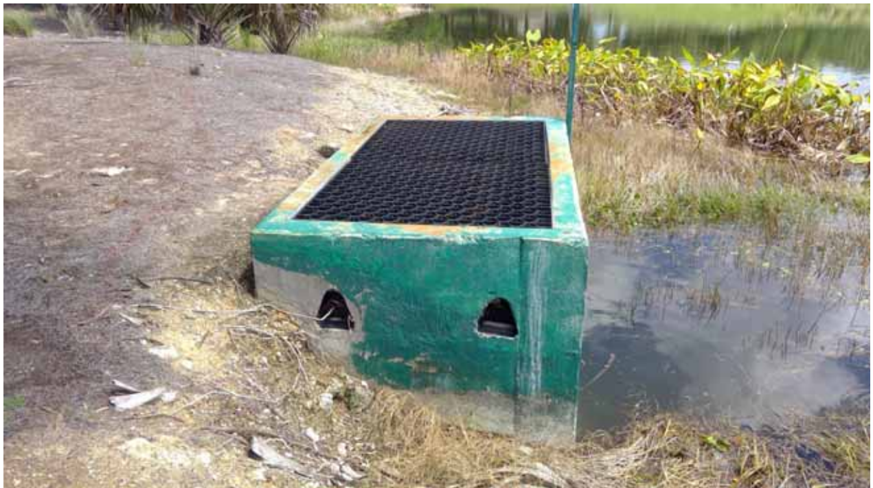
Drainage - Outfall Lake 3A
