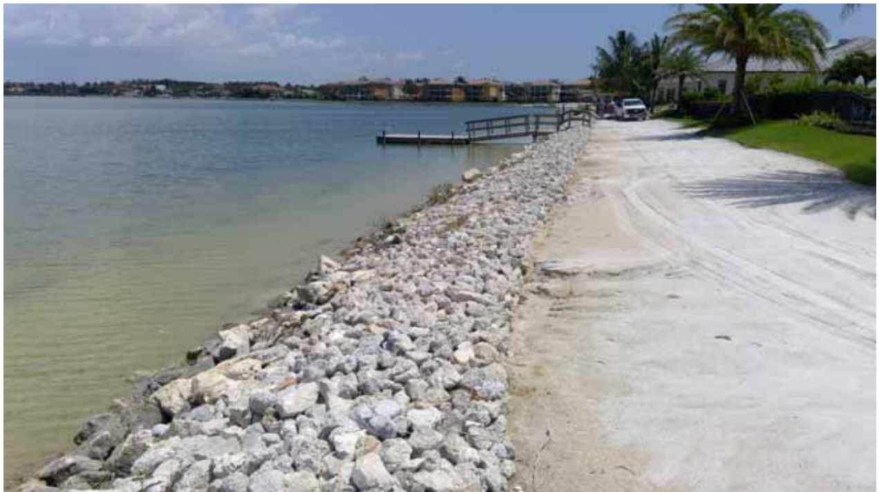
Lake Embankment - 5/6 North
