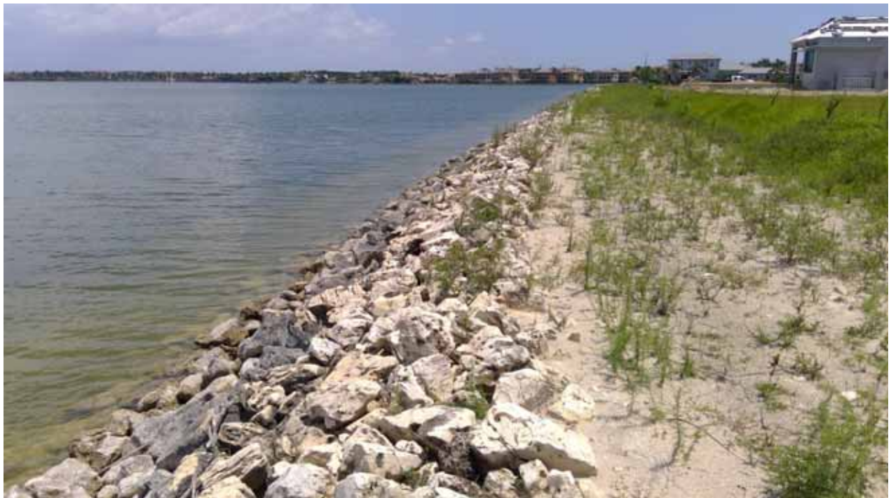
Lake Embankment - 5/6 North
