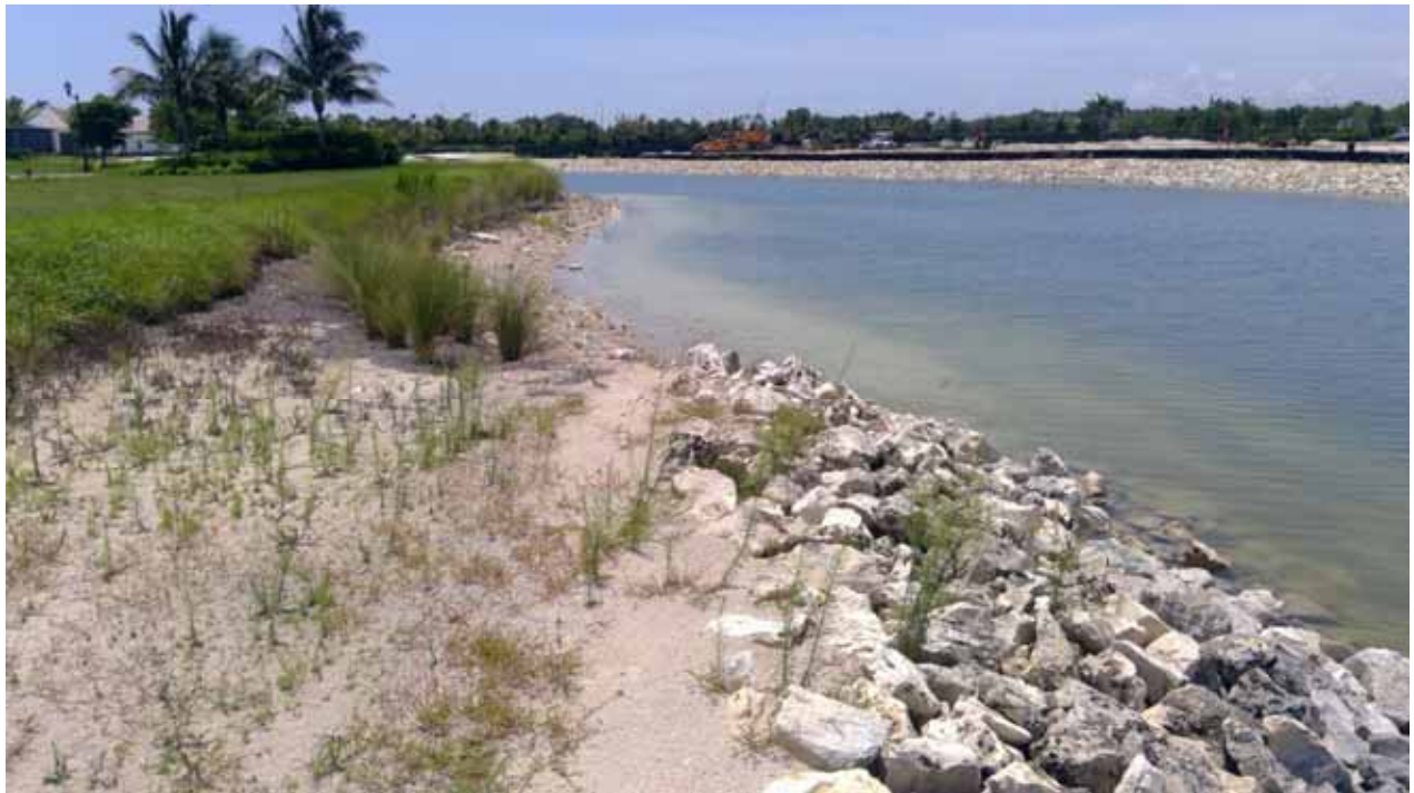
Lake Embankment - 5/6 North
