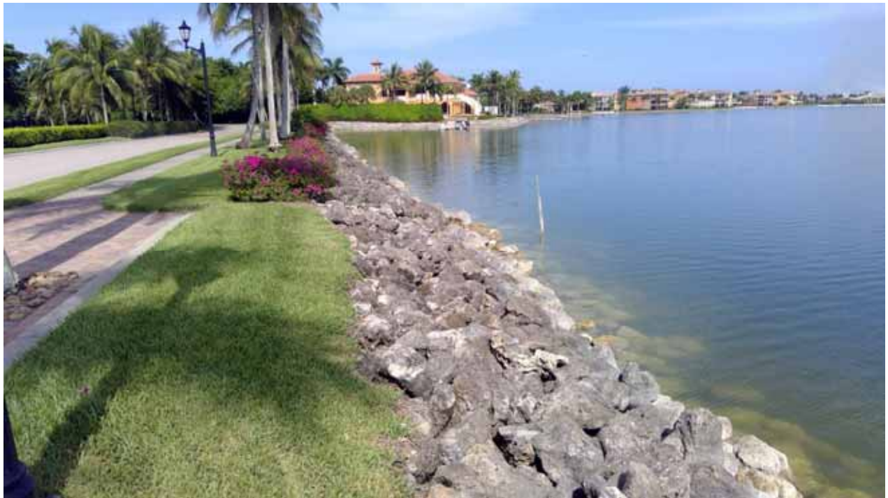
Lake Embankment - 5/6 North
