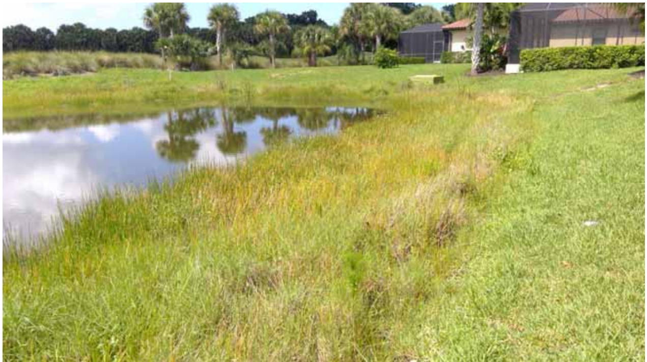
Lake Embankment - 3C
