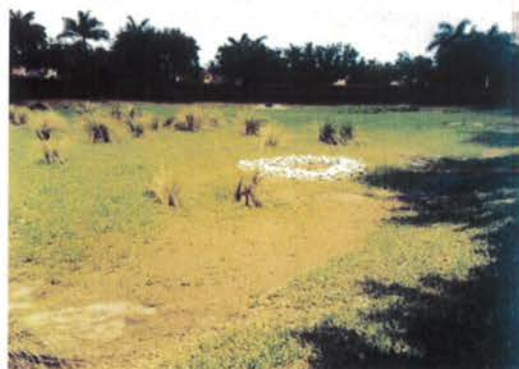
Dry retention areas for stormwater overflow
