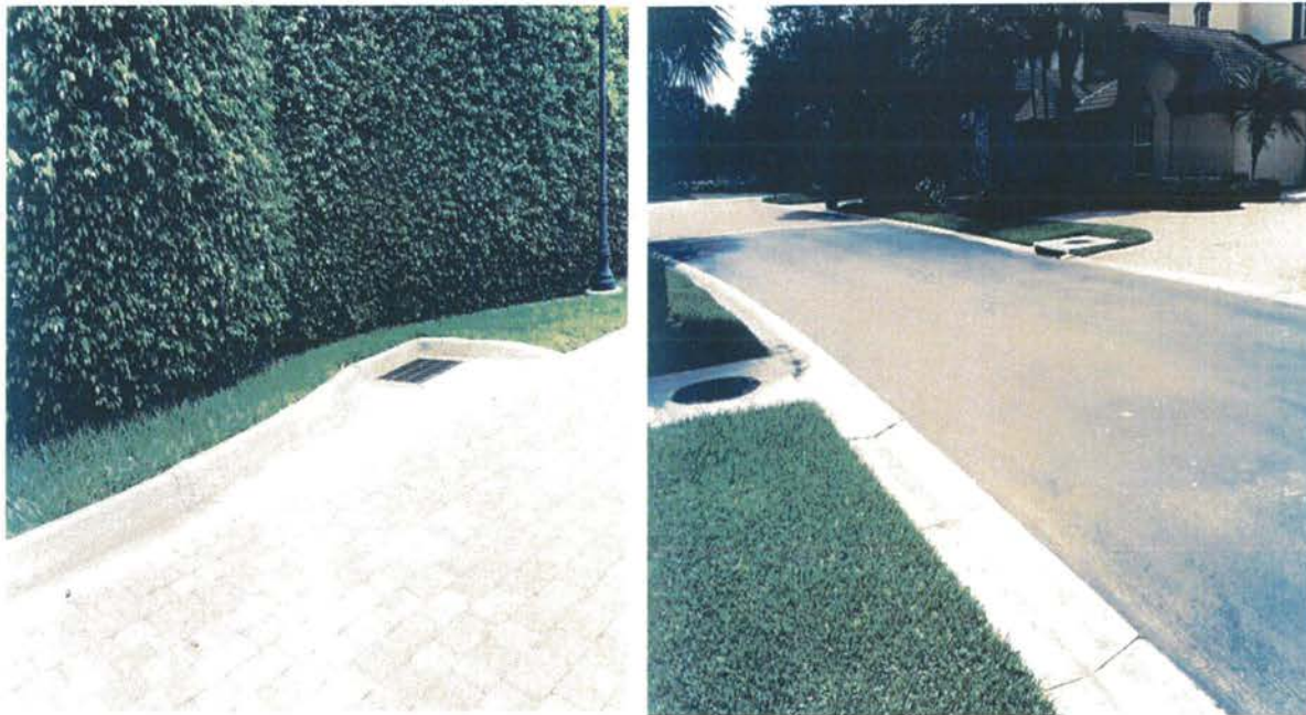
Residential drainage structures for stormwater run-off
