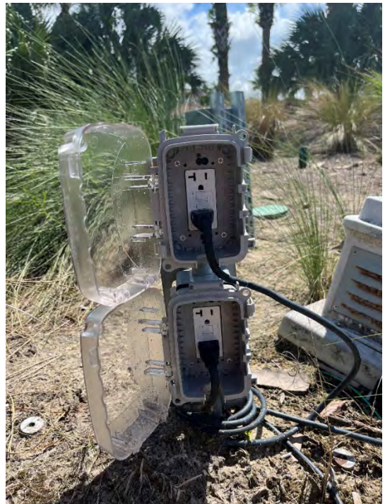
New GFCI reciprocal installed.
