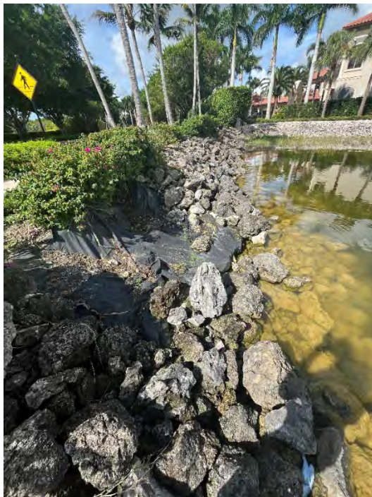
Wash out of the riprap
