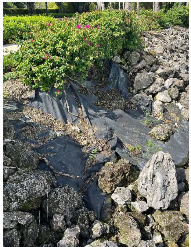
Wash out of the riprap
