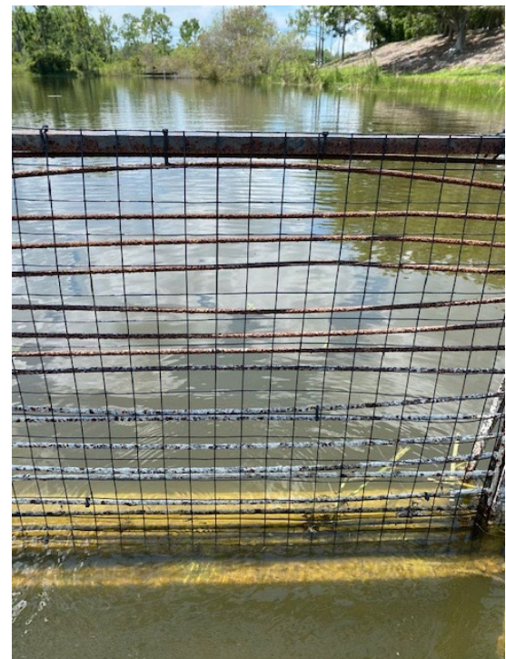
New Fencing Installed at Concrete Weir by FGCU
