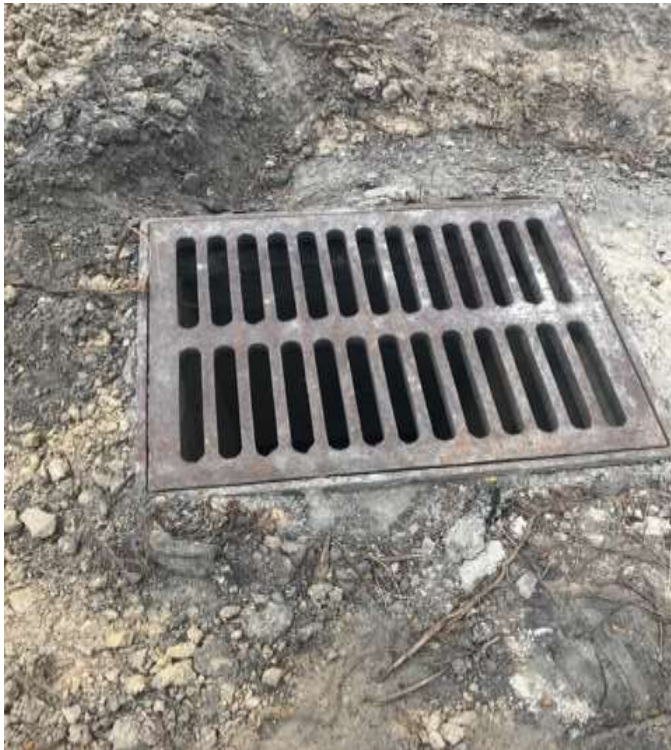
New construction in the parking lot, near the tennis court.
