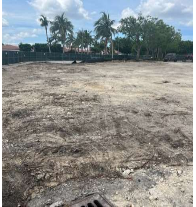
New construction in the parking lot, near the tennis court.
