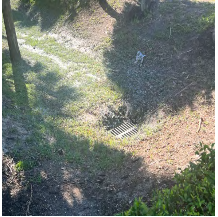
Retention Area Near Volleyball Courts
