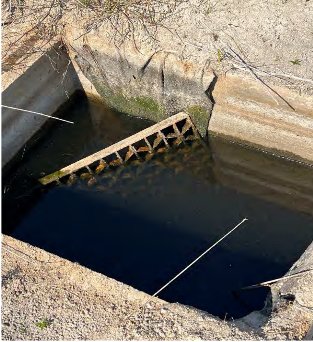
Laguna Catch-Basin Grate
