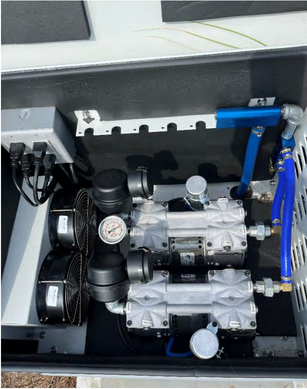
New motor and equipment installed.
