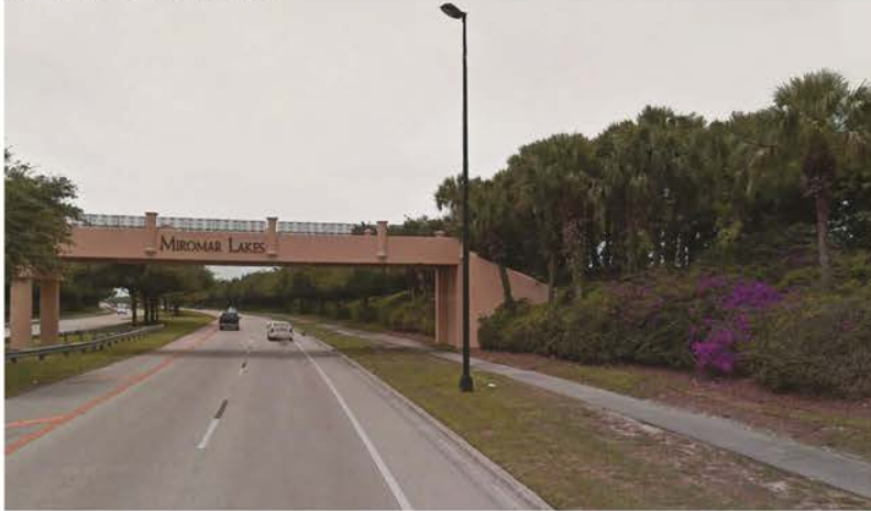
View looking south on west side of bridge.
