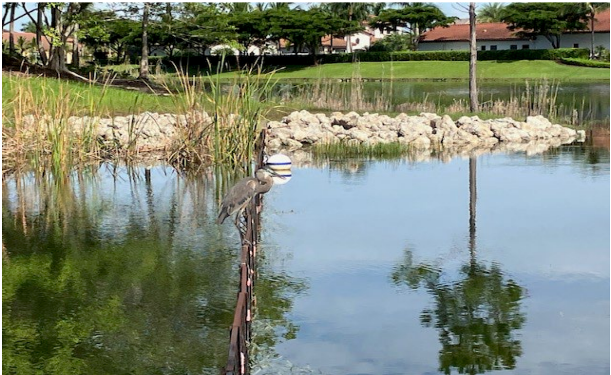
Current conditions at the control weir
