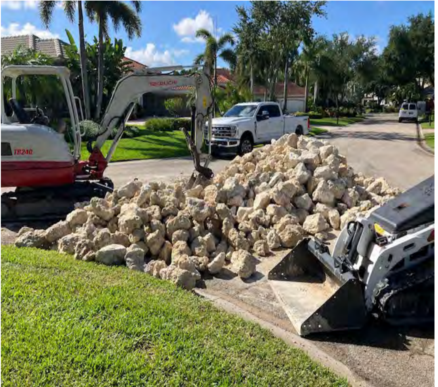
Rip rap installation in progress
