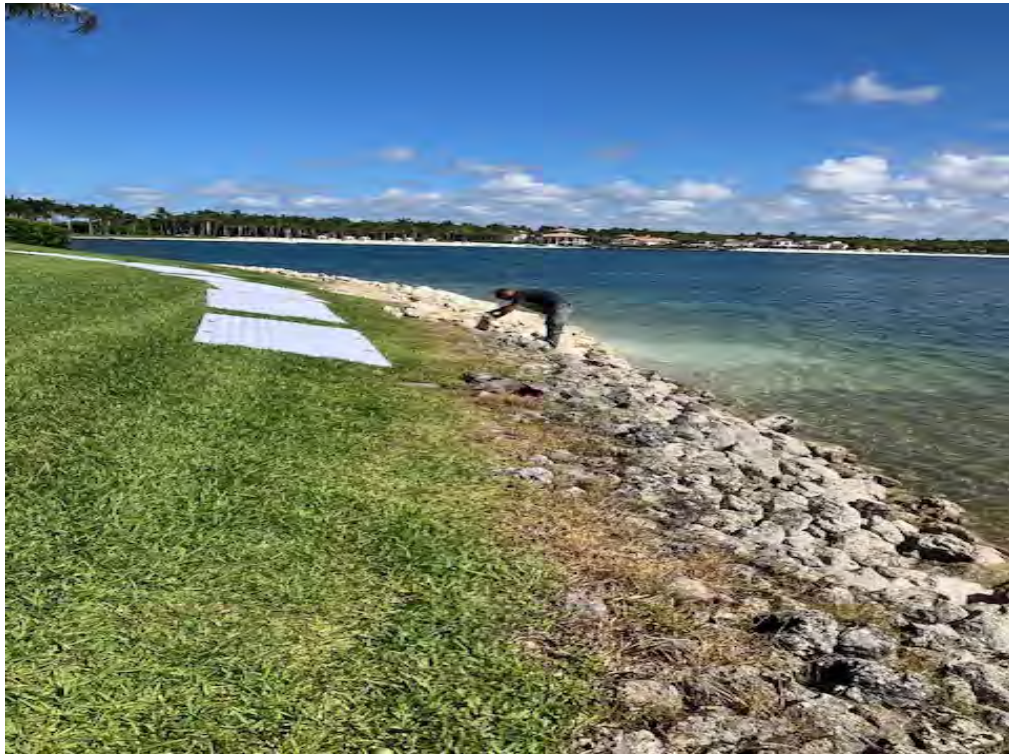
Rib rap installation in progress, with protective materials placed to safeguard surrounding landscaping
