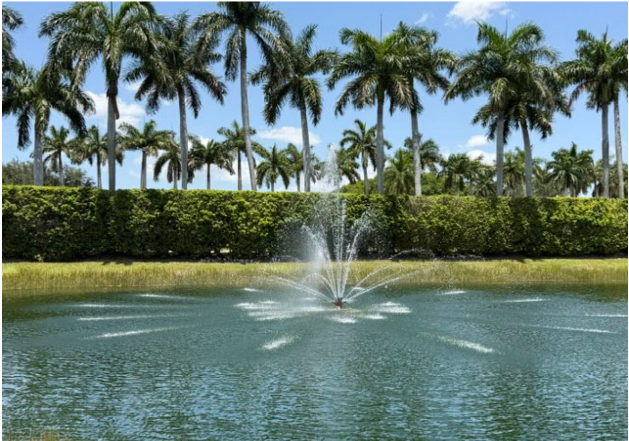
Fountain that Requires Repairs
