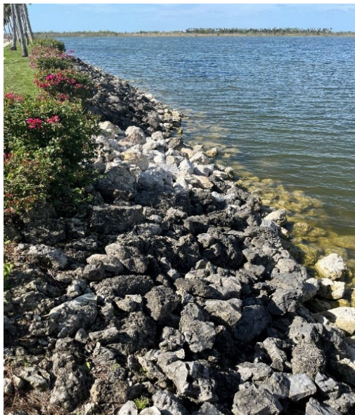
Rip Rap repair completed after hurricane Milton
