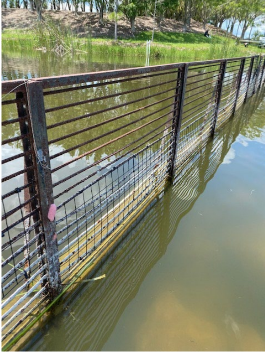
New Fencing Installed at Concrete Weir by FGCU
