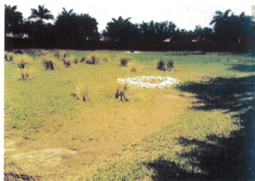
Dry retention areas for stormwater overflow
