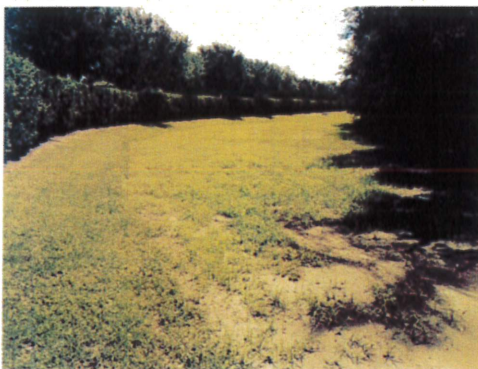
Dry retention areas for stormwater overflow
