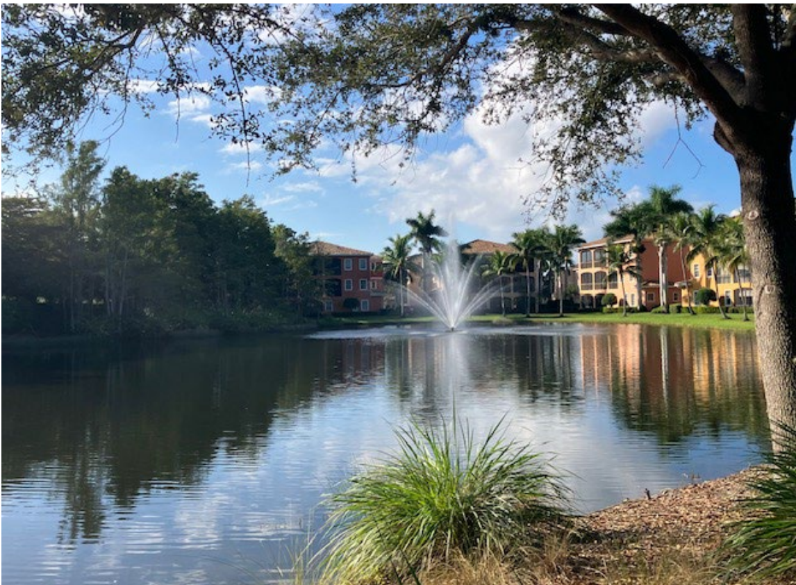
Recently Completed Geotubes
