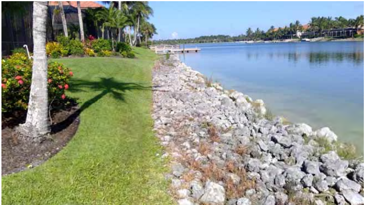
Lake Embankment - 5/6 South
