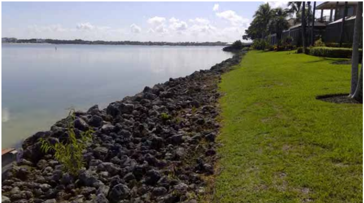
Lake Embankment - 5/6 South
