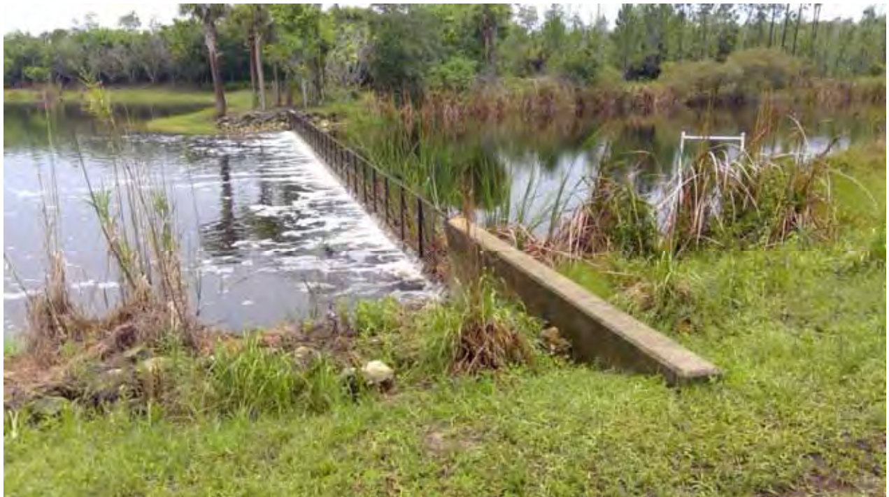
Concrete Weir (FGCU)
