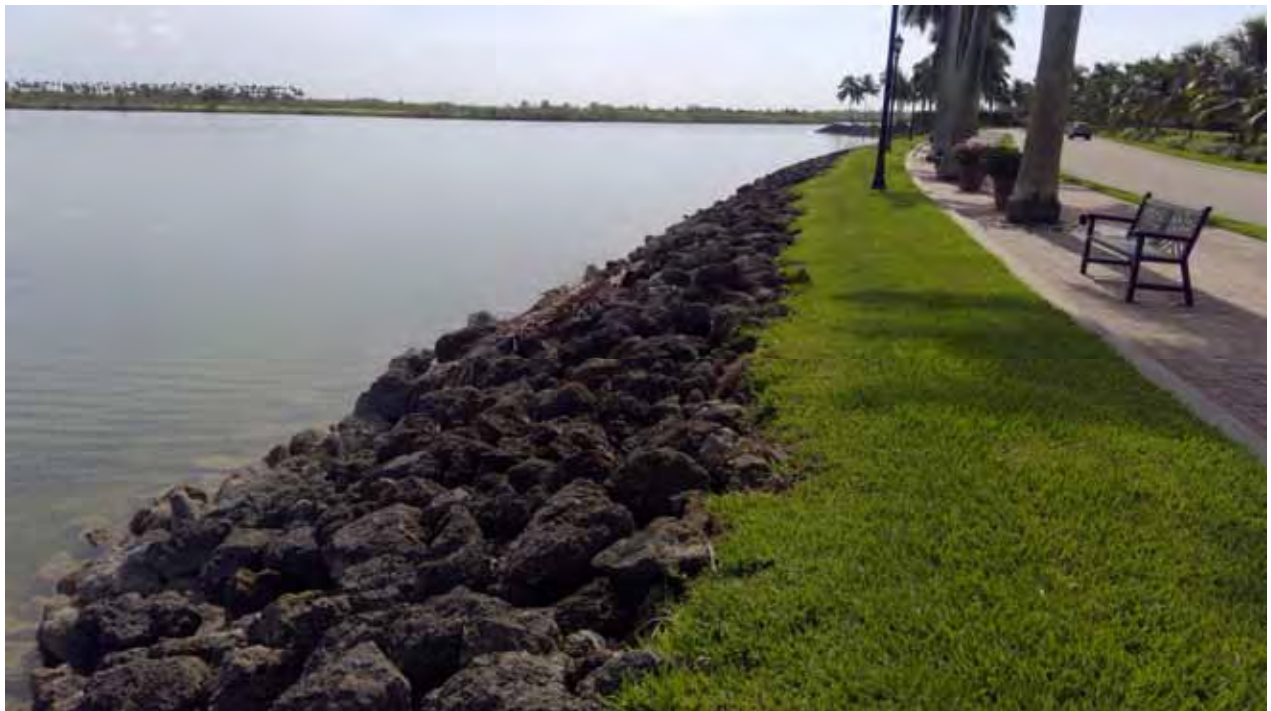
Lake Embankment - 5/6 North
