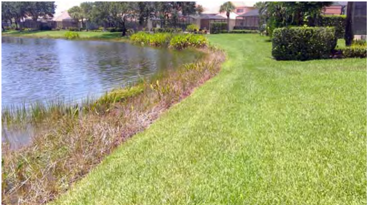
Lake Embankment - 1C
