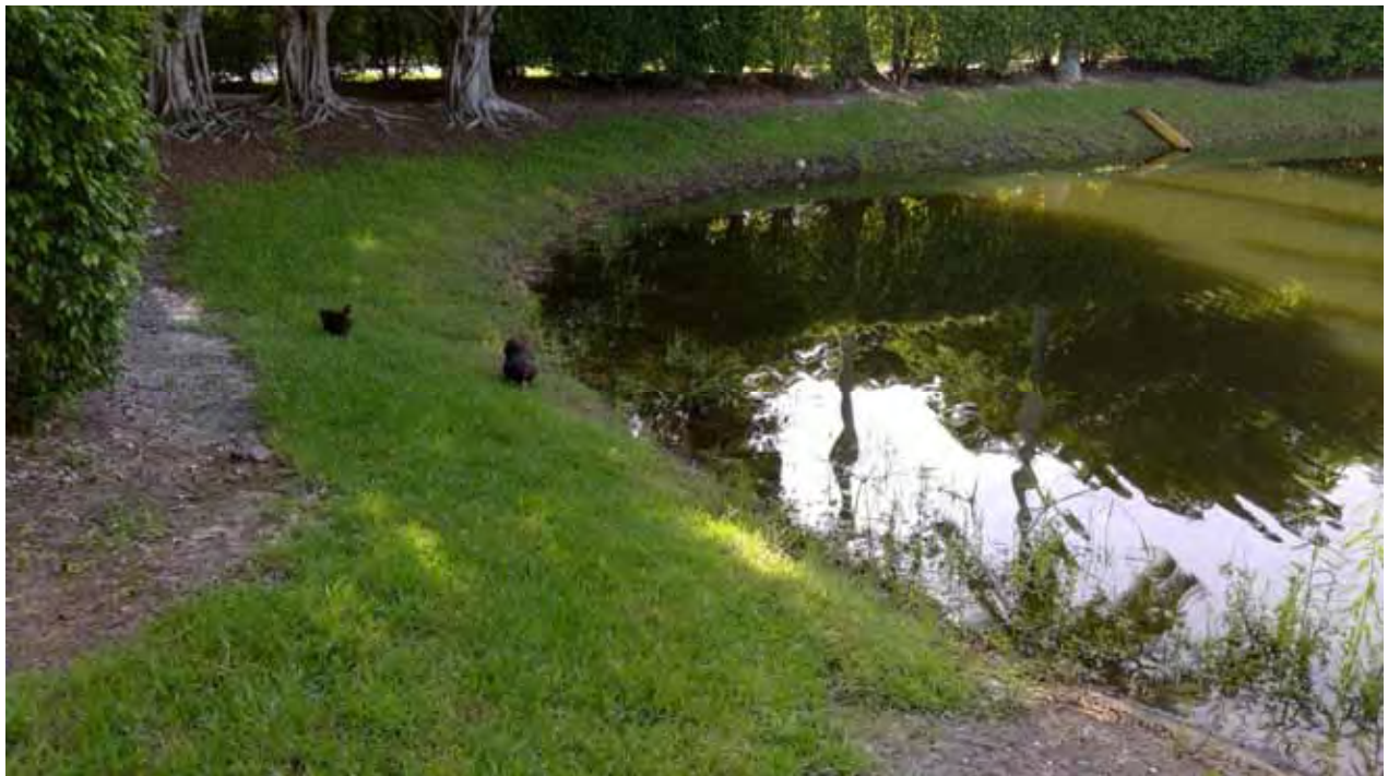
Lake Embankment - 6I
