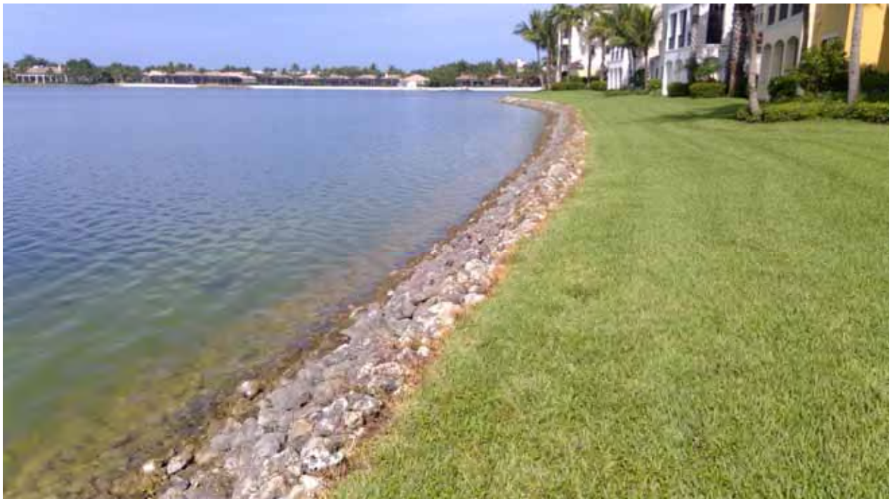
Lake Embankment - 5/6 South
