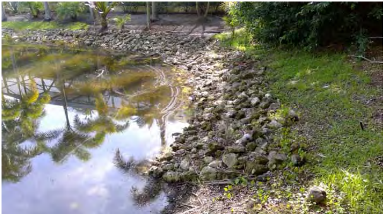
Lake Embankment - Via Bellamare
