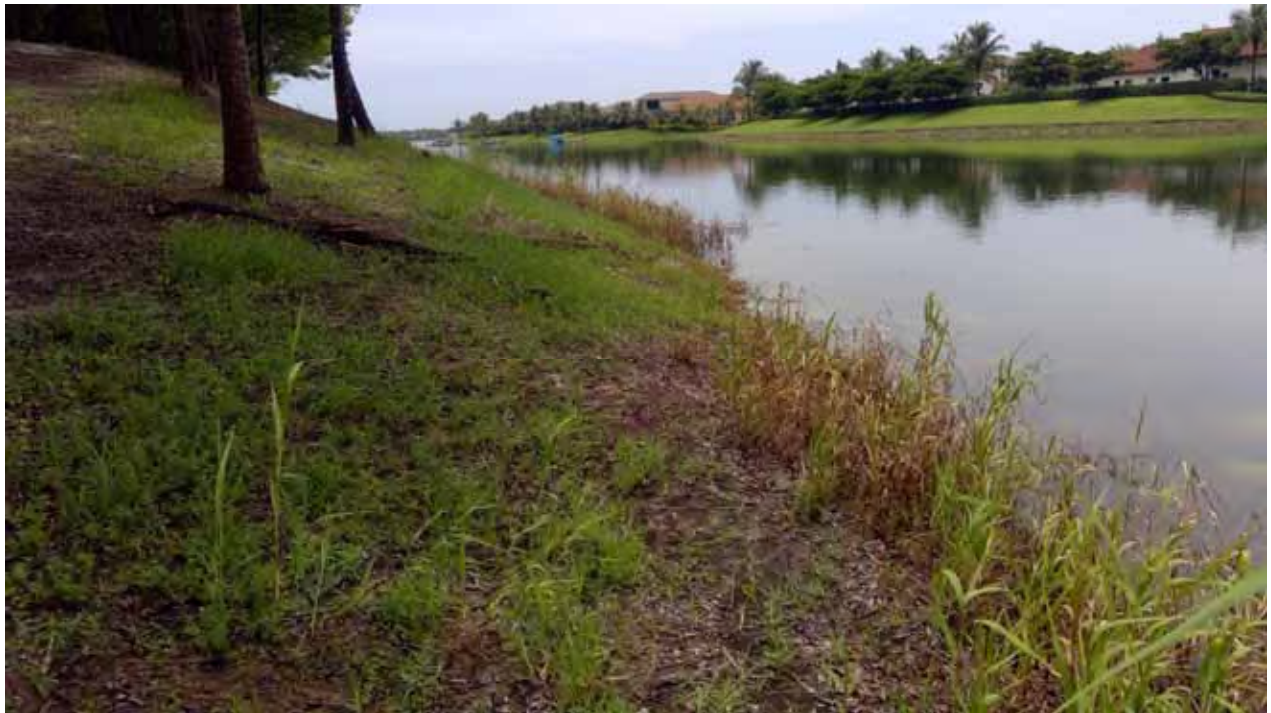
Lake Embankment - 5/6 South
