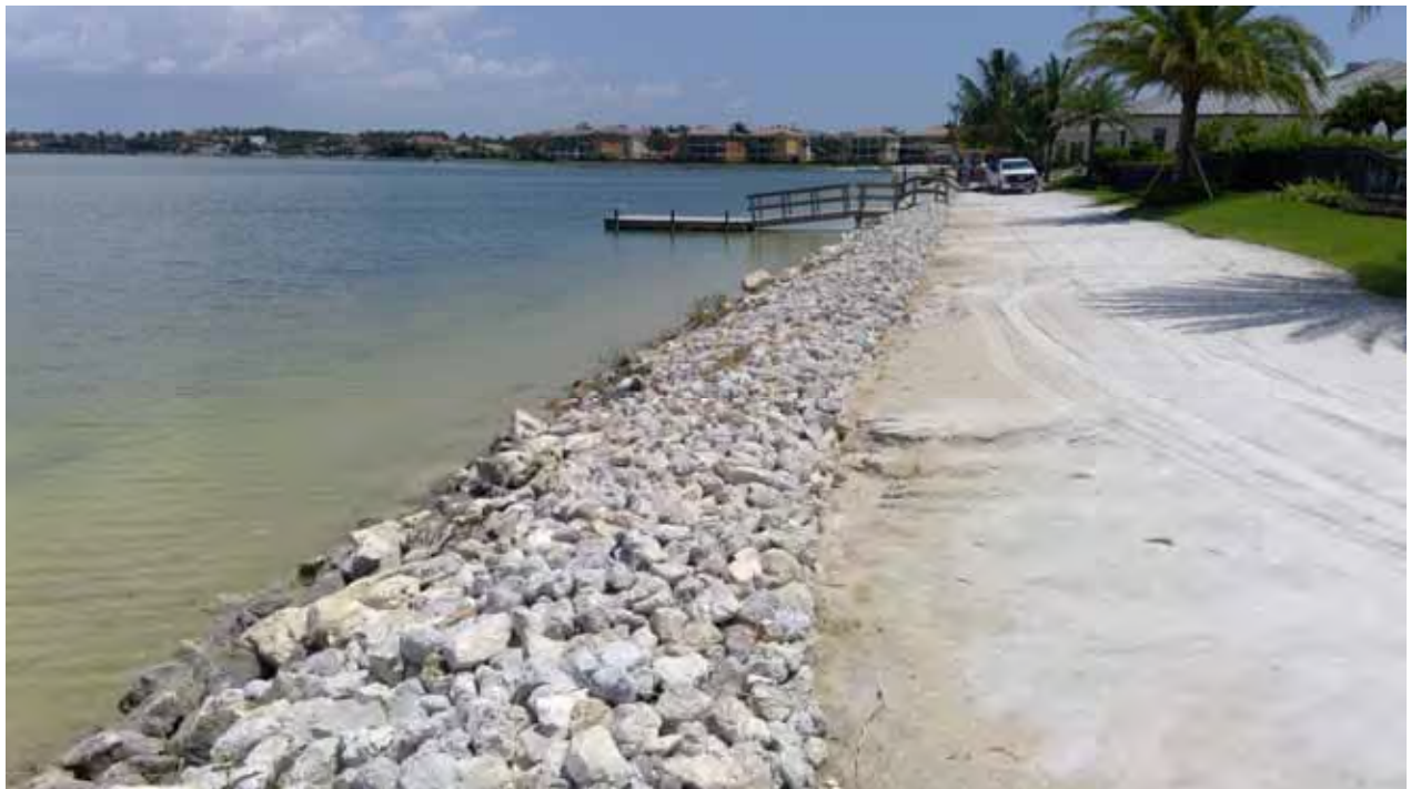
Lake Embankment - 5/6 North
