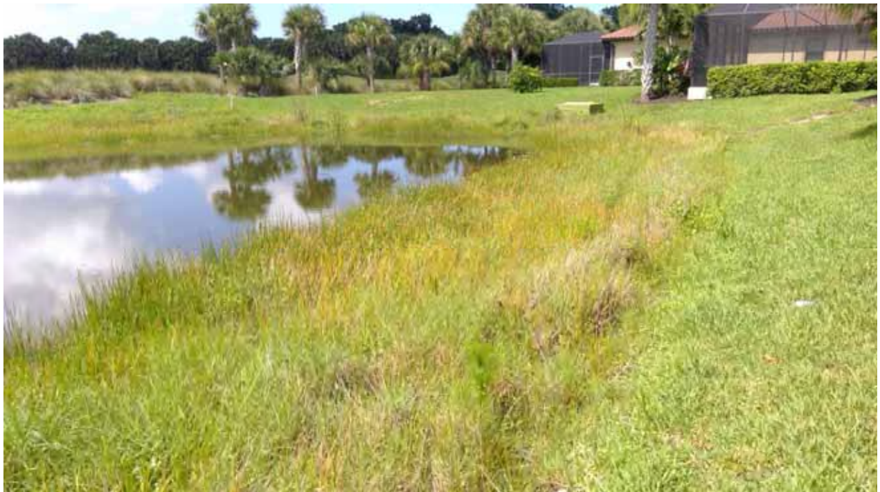
Lake Embankment - 3C
