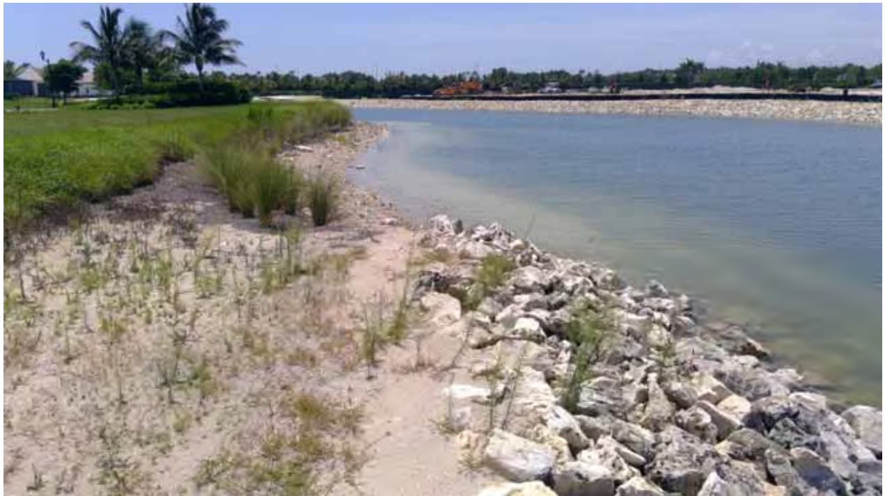
Lake Embankment - 5/6 North
