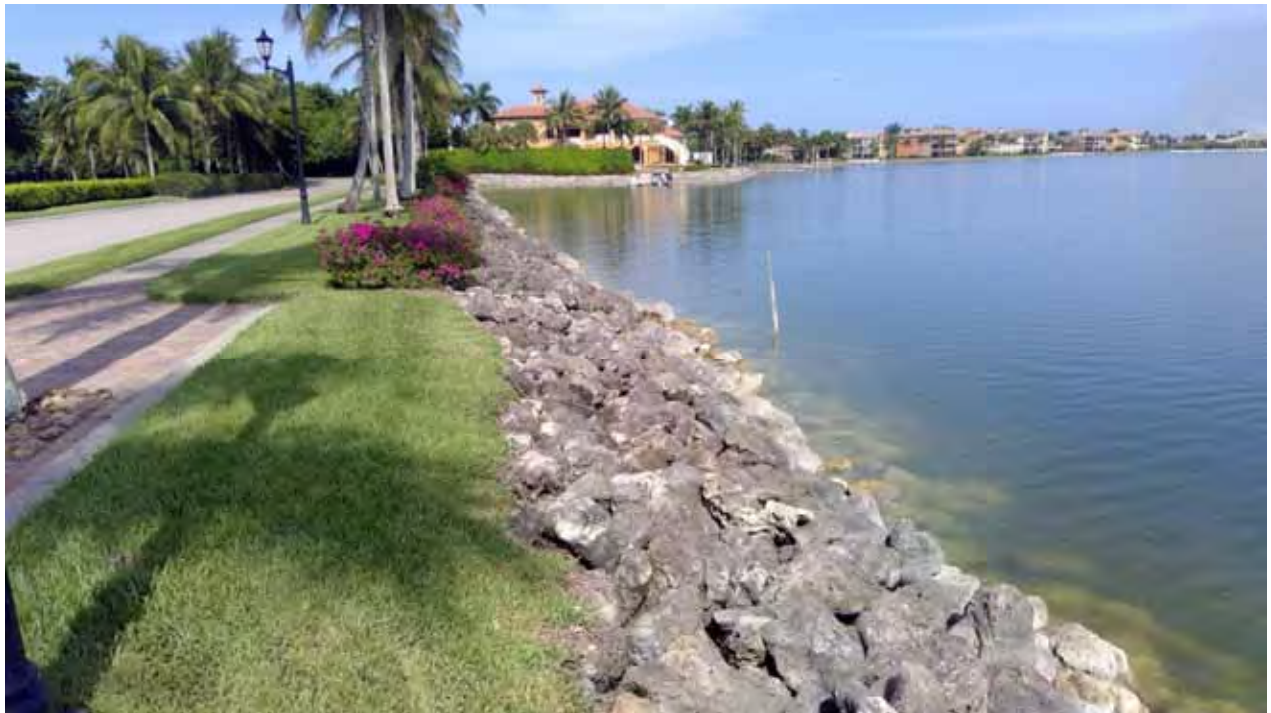
Lake Embankment - 5/6 North
