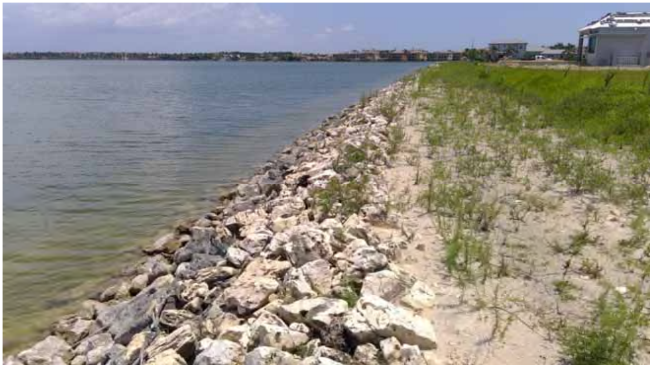
Lake Embankment - 5/6 North
