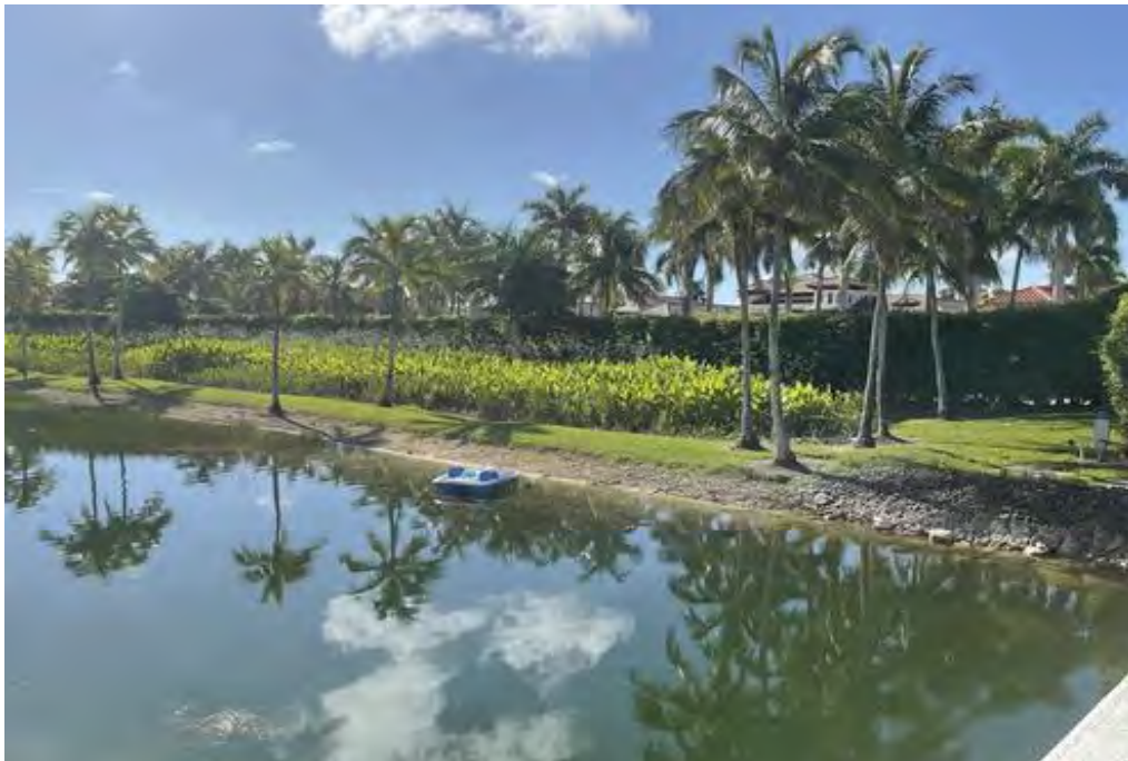
Existing retention pond conditions
