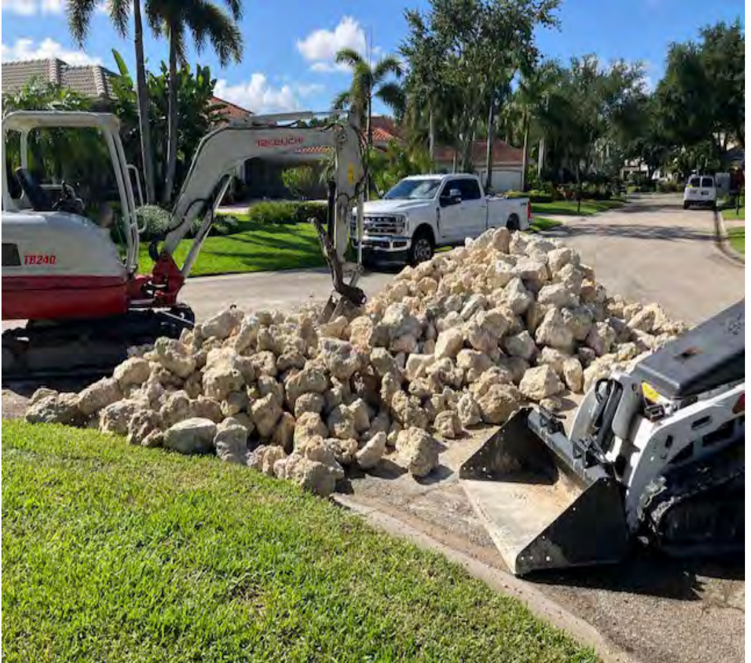
Rip rap installation in progress
