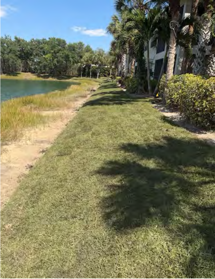
Valencia Lake Bank Completion
