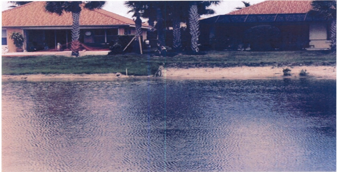
Lake slope after deck installed and adjacent property to east in Porto Romano
