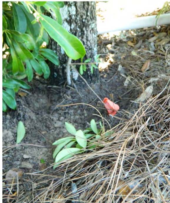
#20 Some Oaks Planted Too Deep
