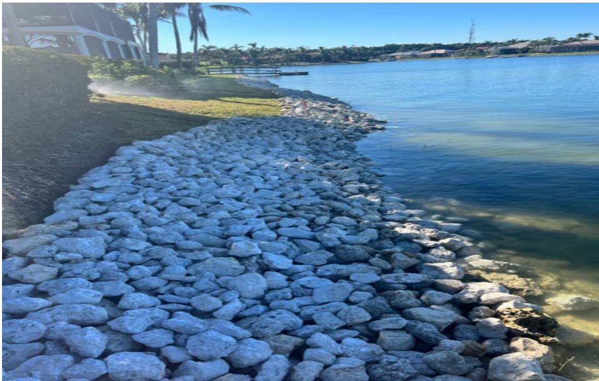
RIPRAP INSTALLATION AND ISABELLA
