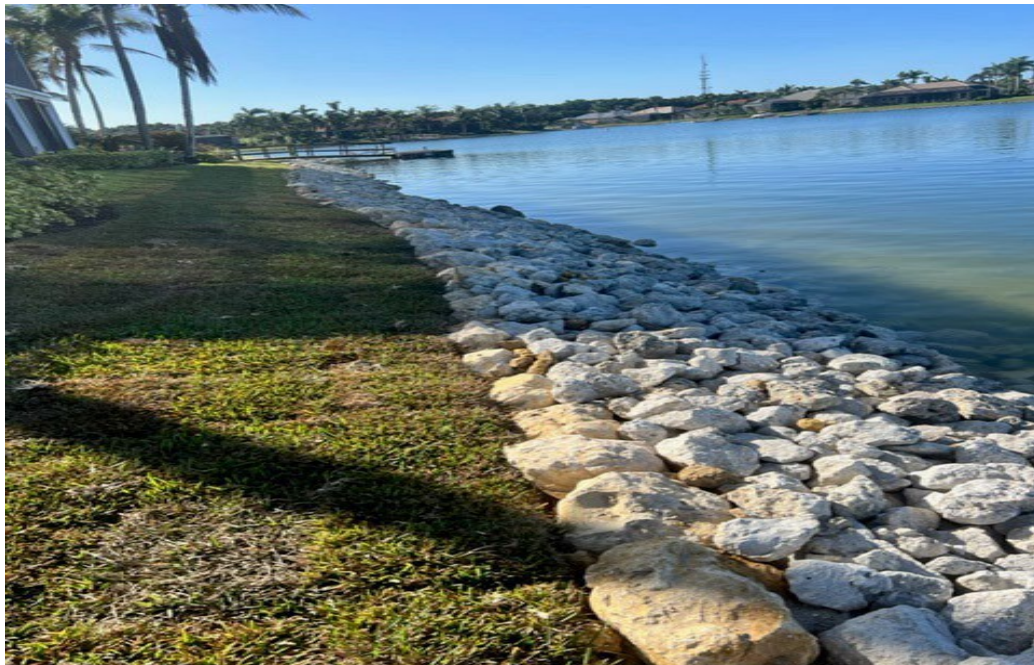
RIPRAP INSTALLATION AND ISABELLA
