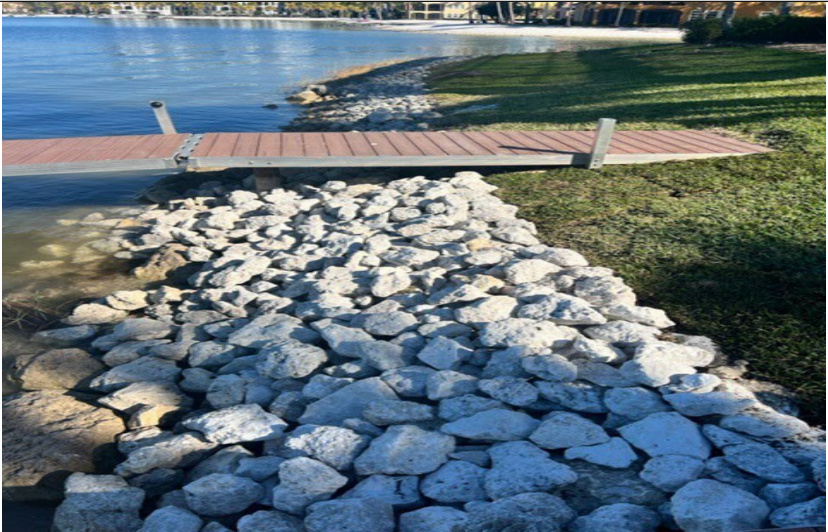
RIPRAP INSTALLATION AND ISABELLA
