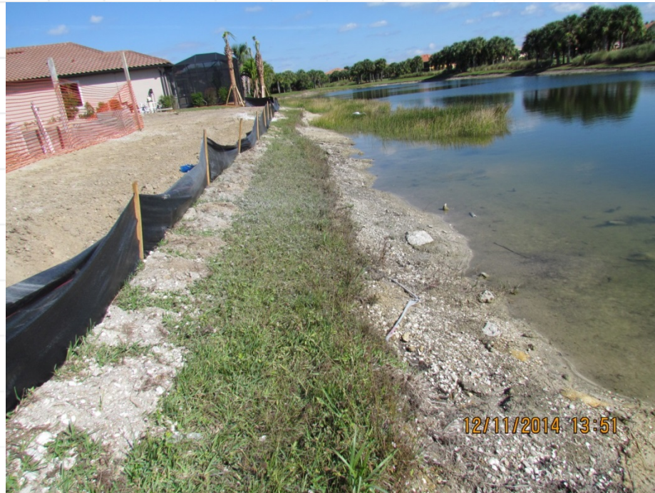
Figure 3- San Marino South Lake bank in Dec. 2014
