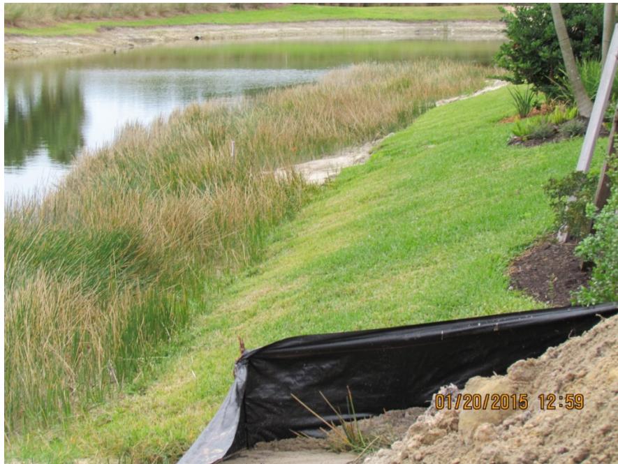
Figure 2- WCI completed bank slope construction on San Marino South Lake Jan. 2015
