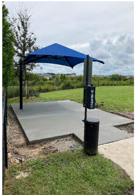
New dog park concrete pad
