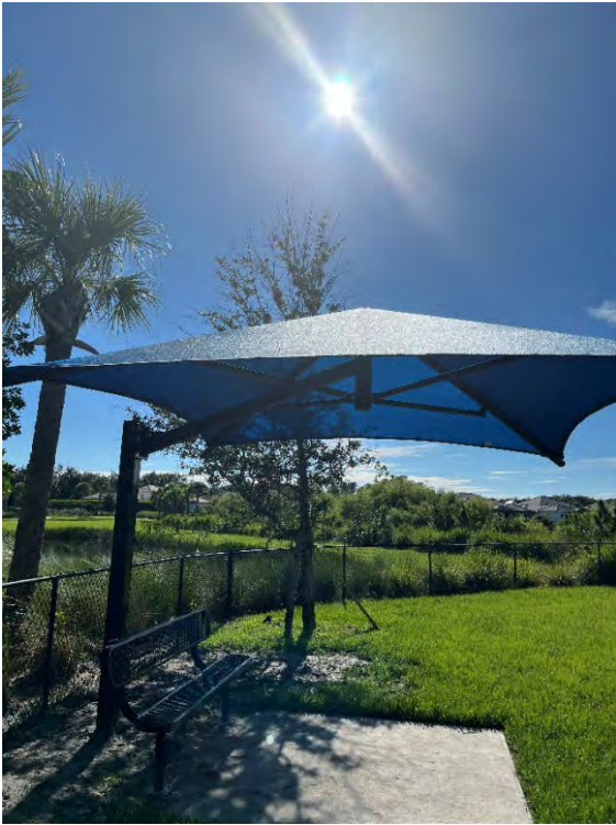
New shade structures installed at the dog park.
