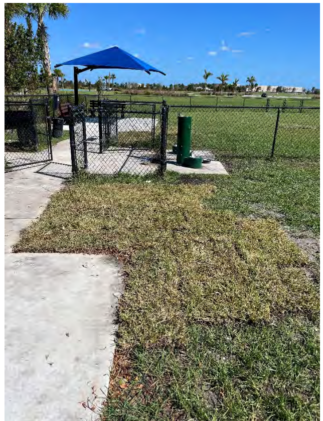
Sod installed around new concrete pads.
