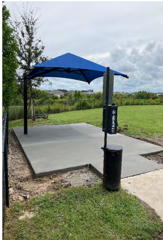
New dog park concrete pad.
