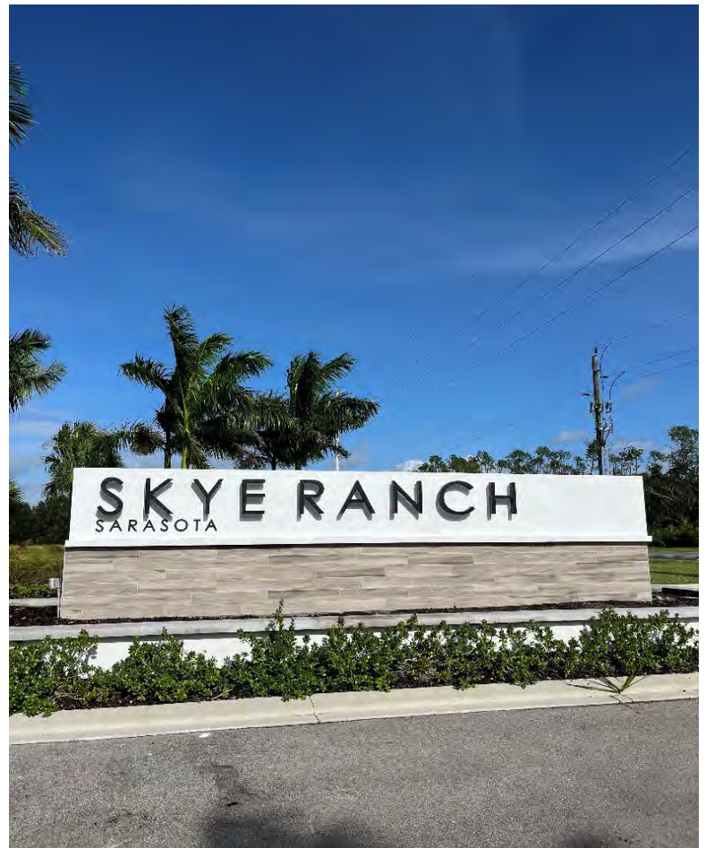
Monument on Night Skye Ave was repaired
