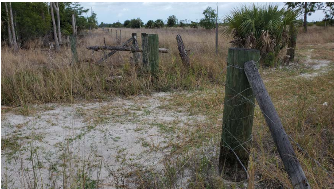
Flow Way CDD Gate 2 – Broken
