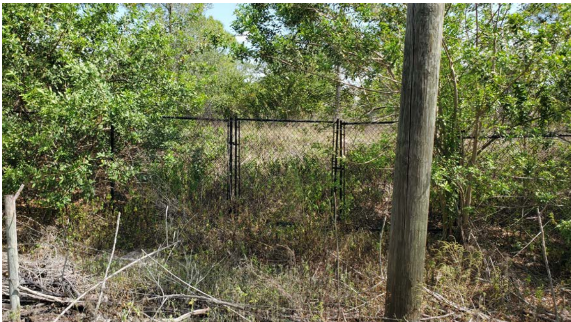
Village Walk of Bonita Springs – Chain link fence (others)
