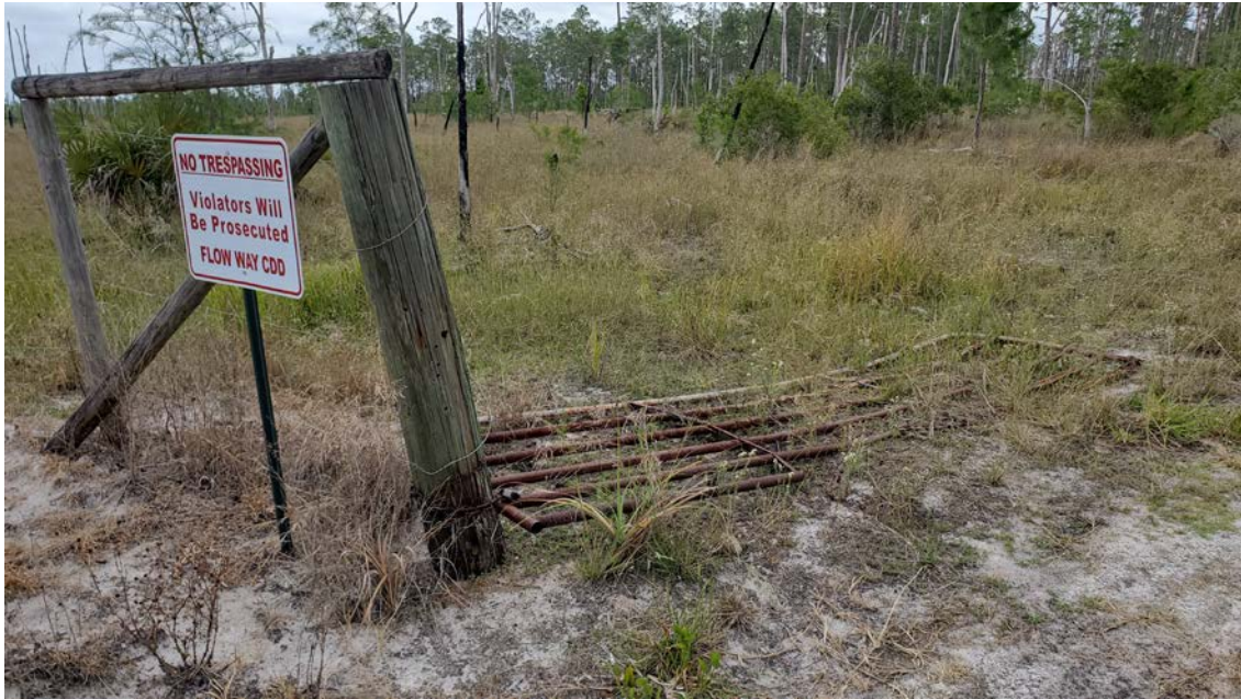
Flow Way CDD Gate 1 – Broken
