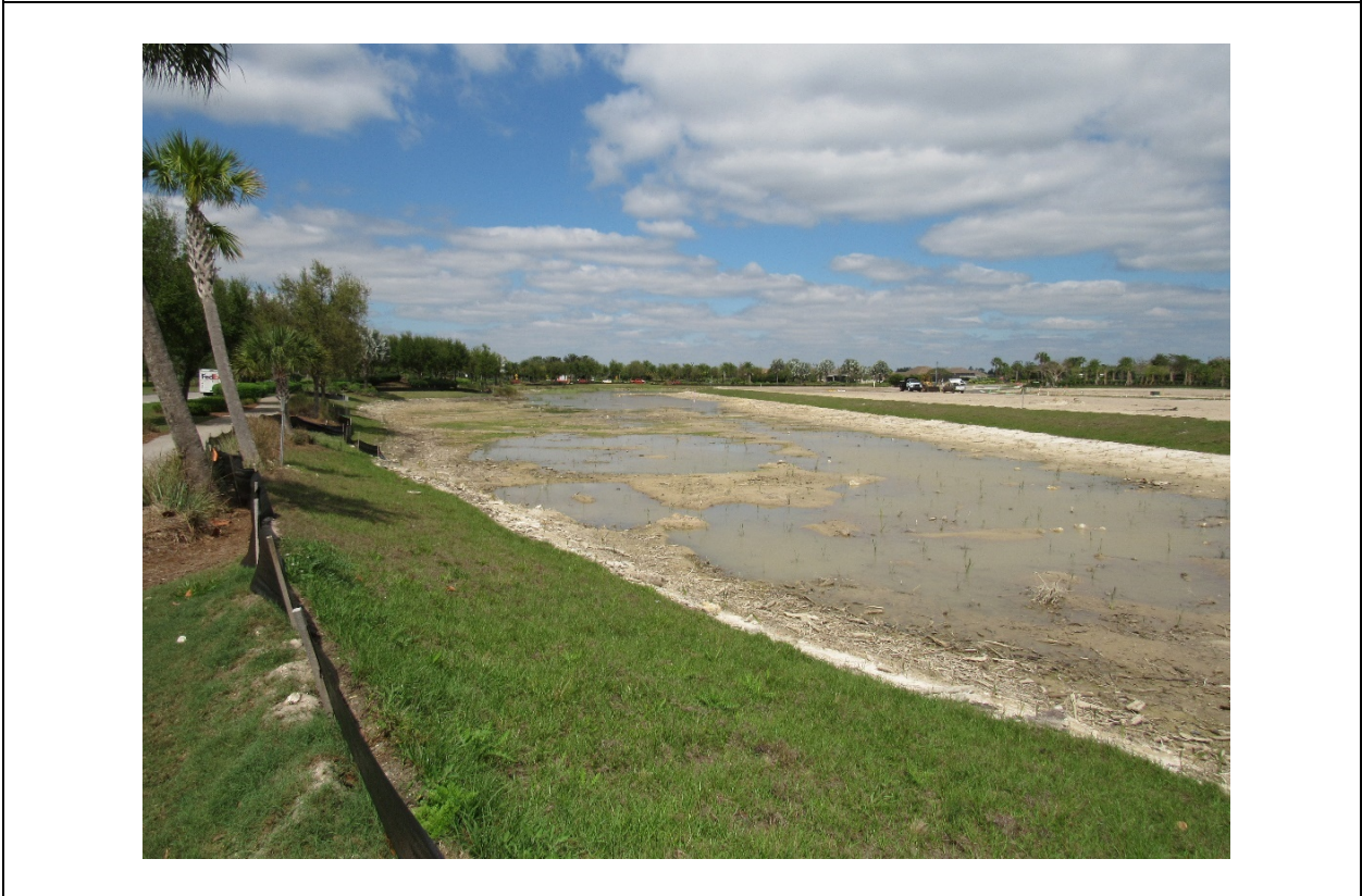
View of lake under construction - Lake 11.
