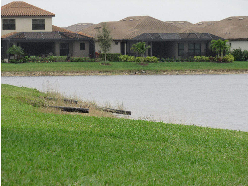
Typical view of limited littoral plants and direct discharge lines - Lake 18.
