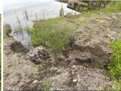
Large washout needs attention
