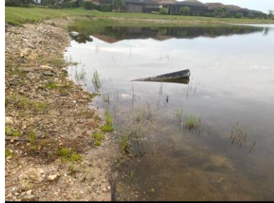
Pipe not anchored down
