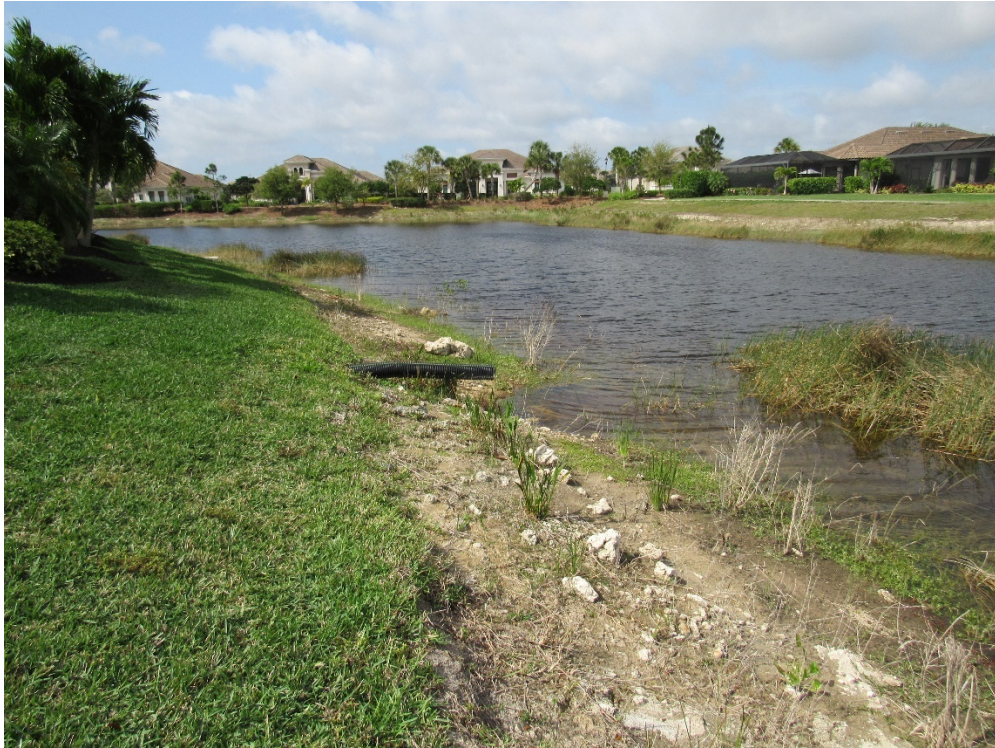
View of erosion at discharge line - Lake 14.
