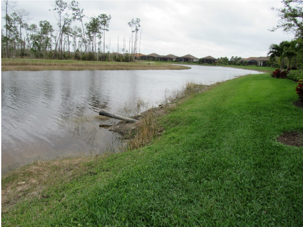
View of erosion at lake embankment - Lake 18.
