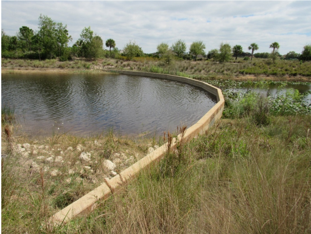
View of South Broad Crested Weir.
