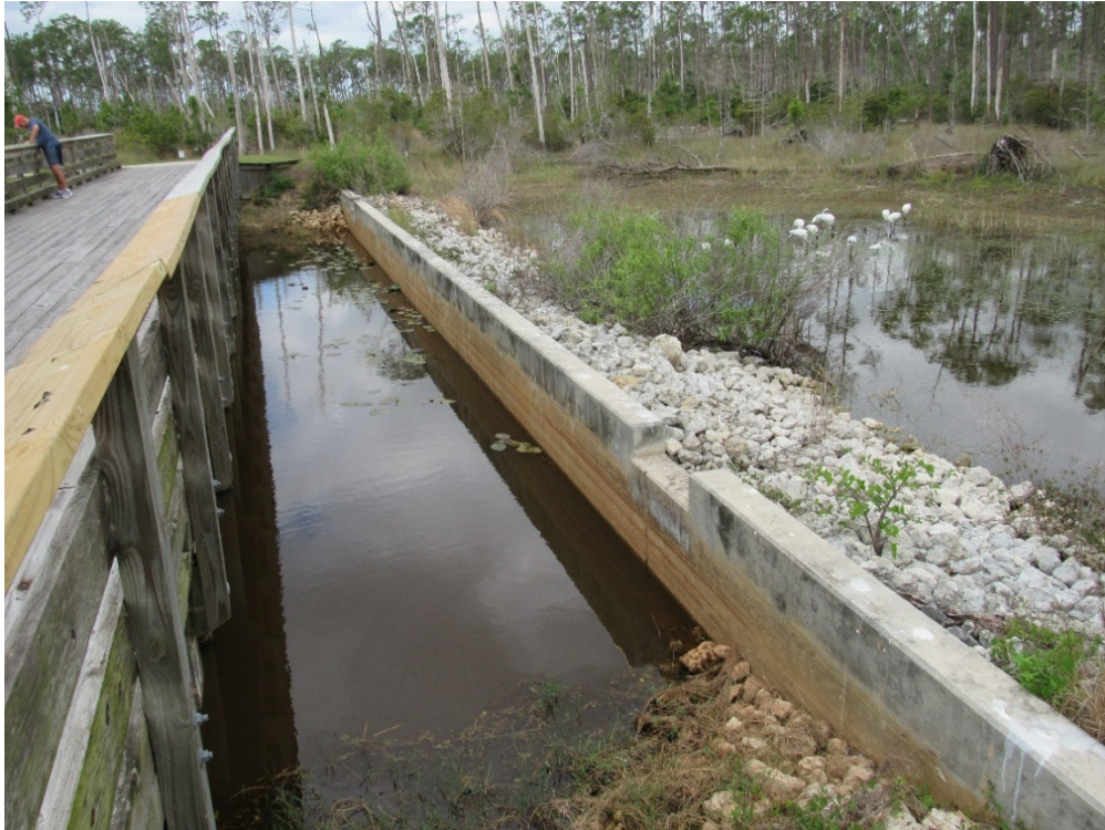
View of North Broad Crested Weir.
