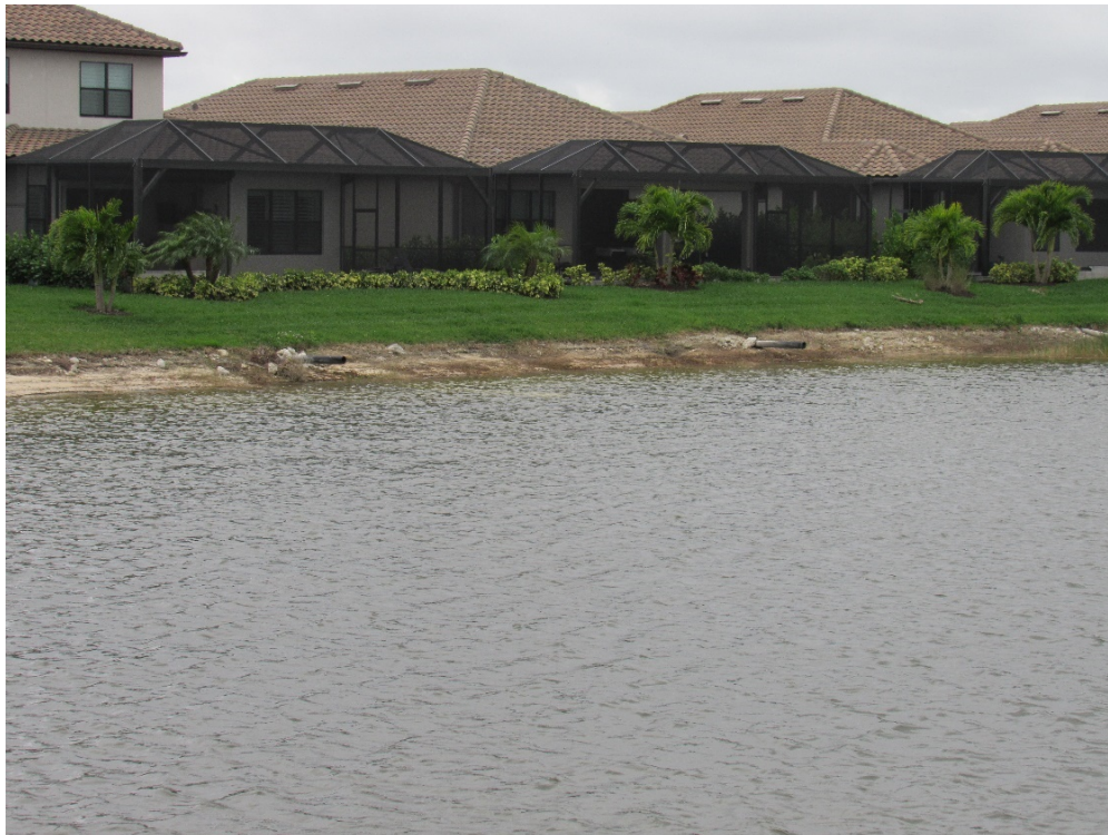
Typical view of limited littoral plants and direct discharge lines - Lake 20.
