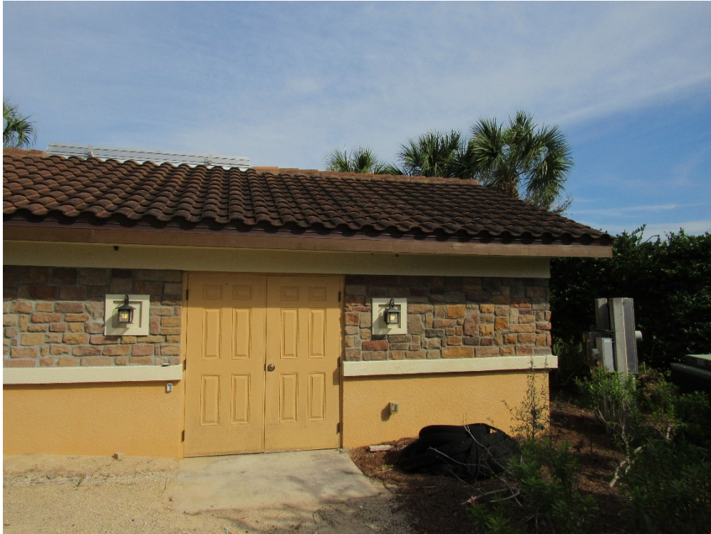
Exterior view of Community Irrigation Pump House.
