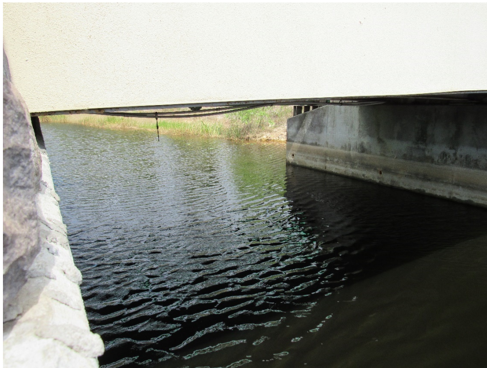
View of Flow Way at intersection with Immokalee Road Canal.
