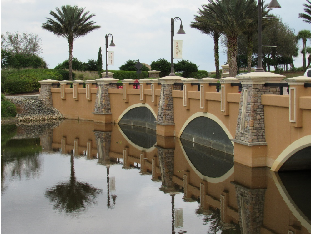
View of Entry Bridge
