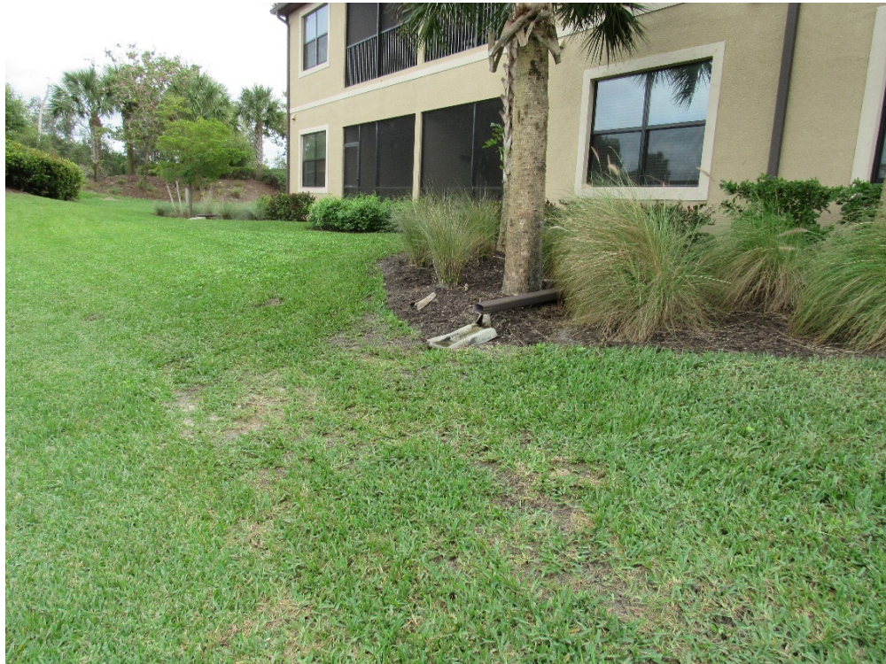
View of gutter downspout from a building - Lake 17/Benvenuto Court.
