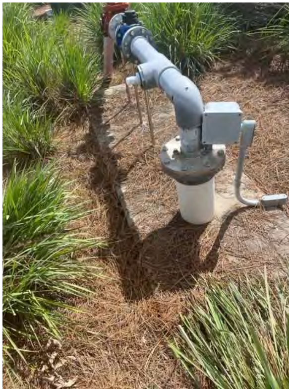
Irrigation - Recharge Well - Hole 12
