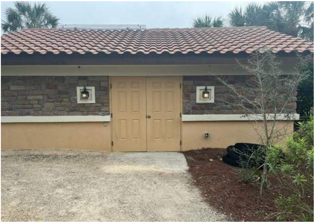
Irrigation - Pump House (External)
