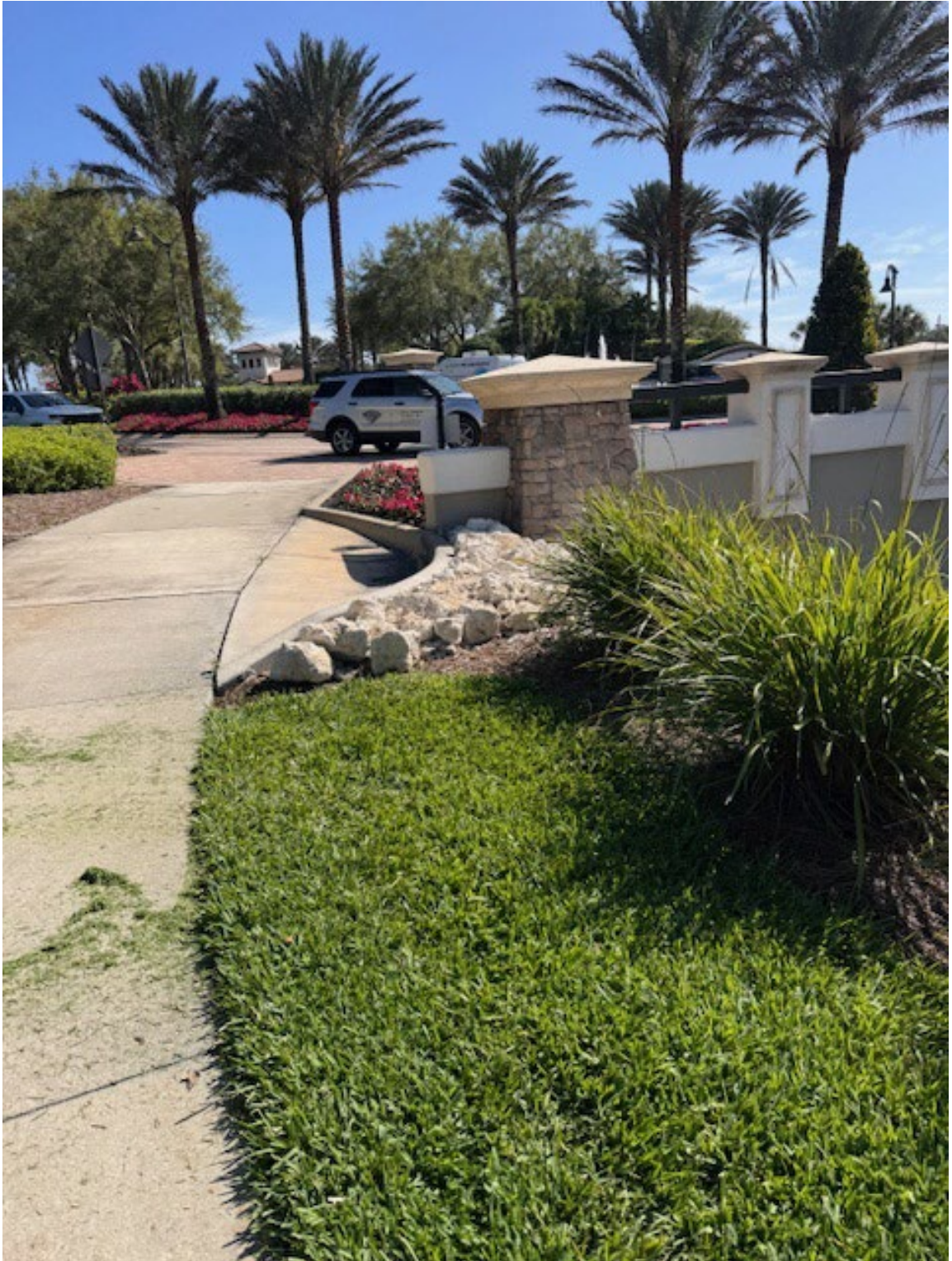
(8) New Rip-Rap on NW side of bridge
