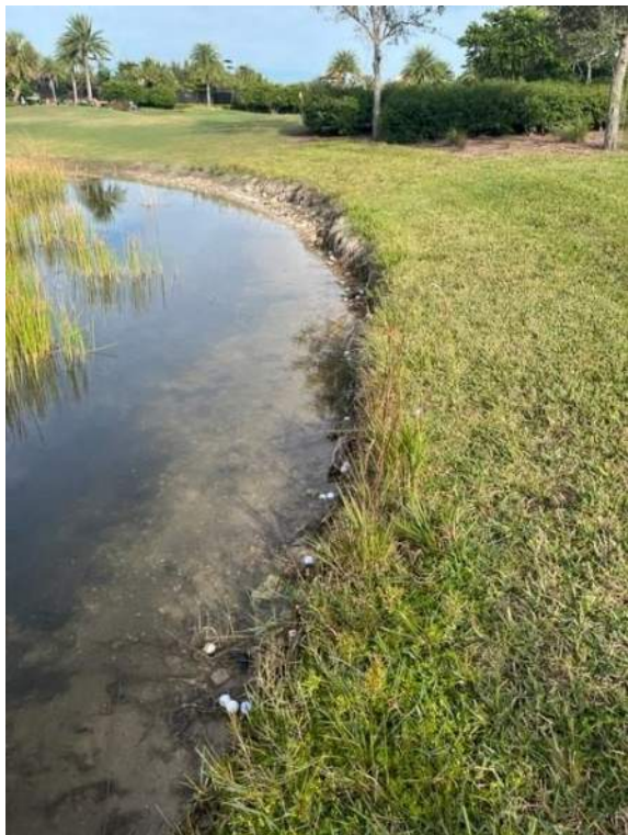
SWM - Lake Bank Slope (Aqua Range)
