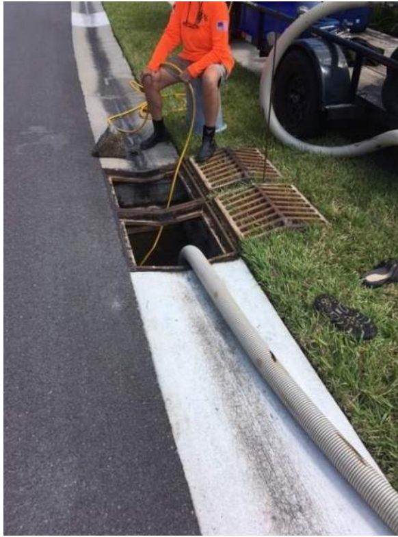
SWM - Drainage Structure
