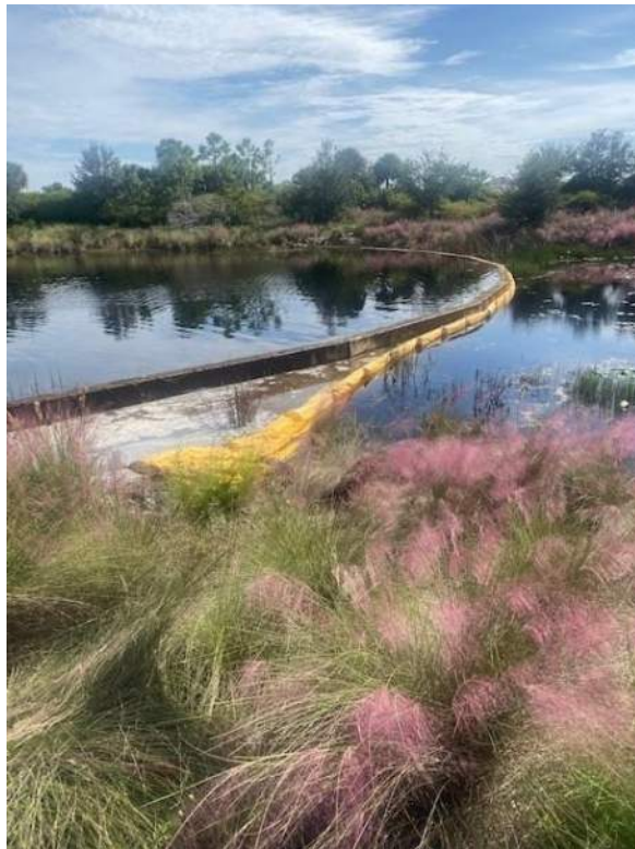
SWM - Flow Way Weir (South)
