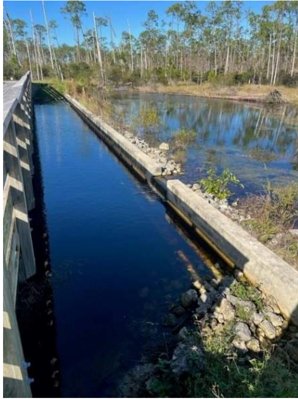
SWM - Flow Way Weir (North)
