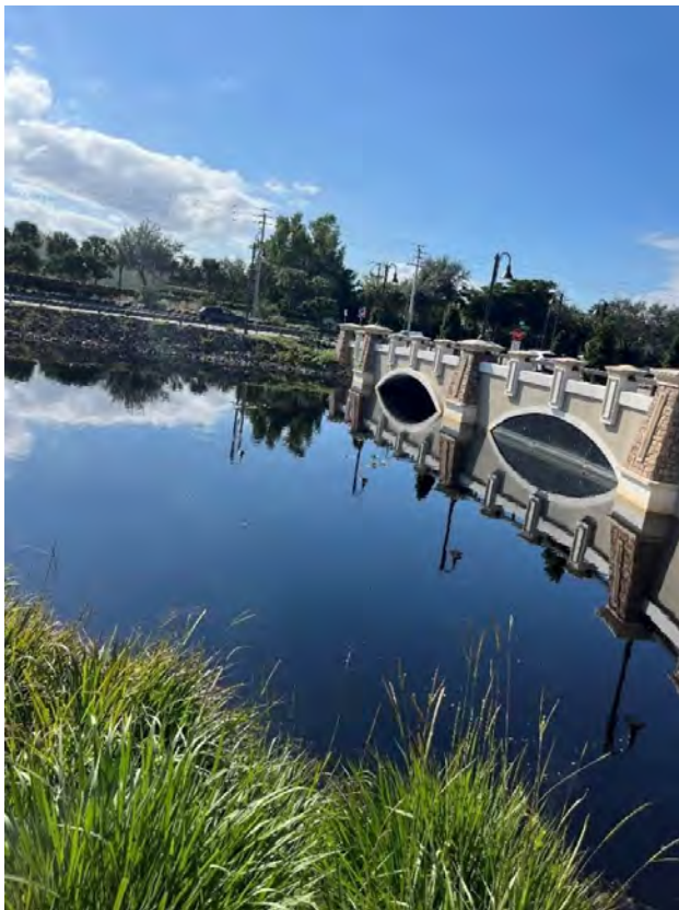
(6) Immokalee Canal debris cleaned by SFWMD/ Collier County
