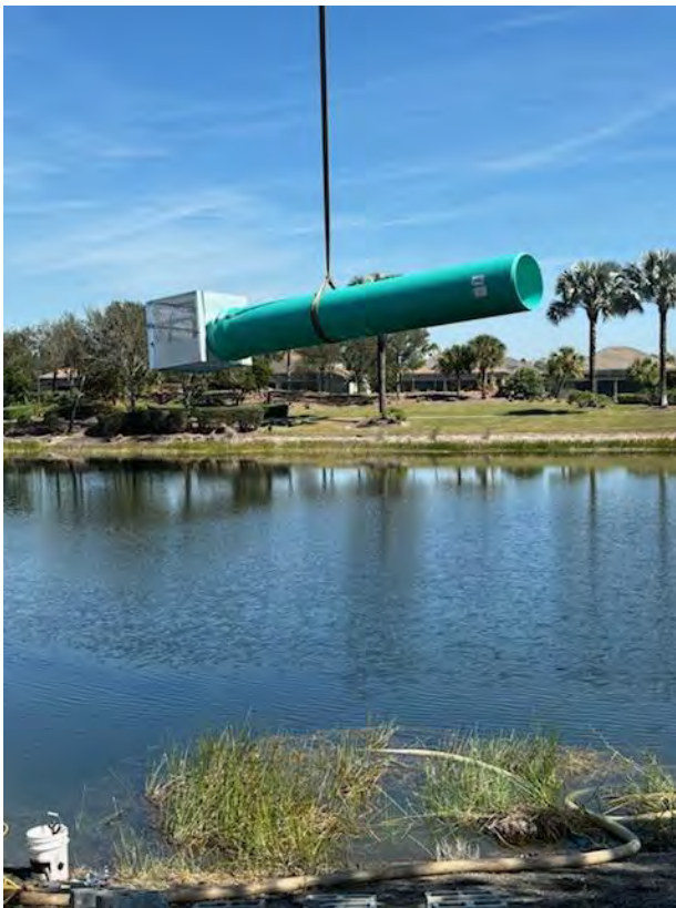
(13) Intake Pipe instaling at Pump House
