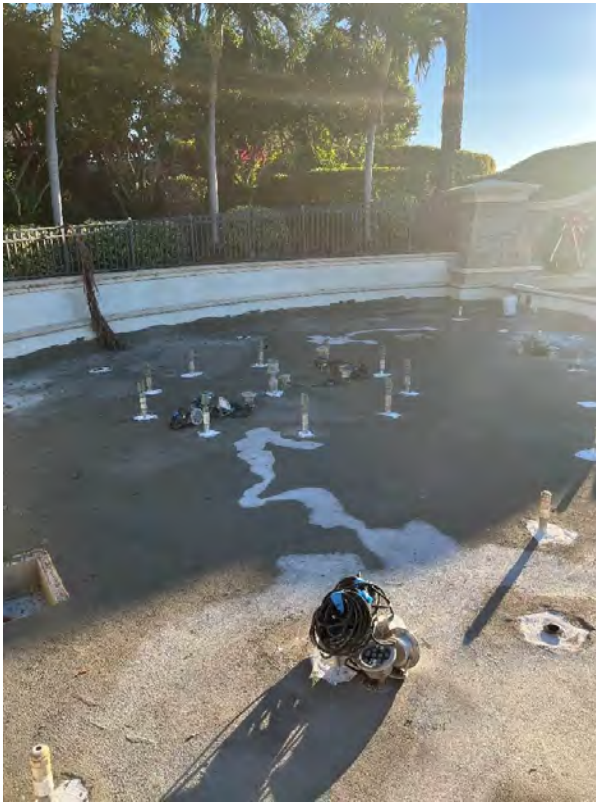
(7) Fountain Diamond Brite under construction
