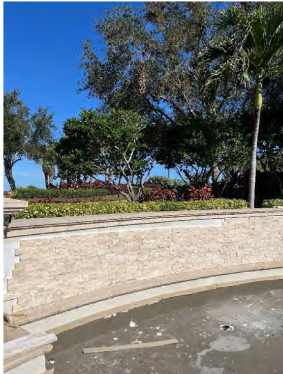
(10) Fountain under Construction
