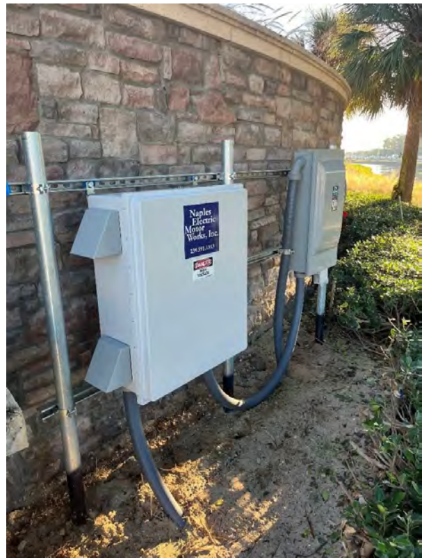
(8) New Fountain Electrical Panel installed
