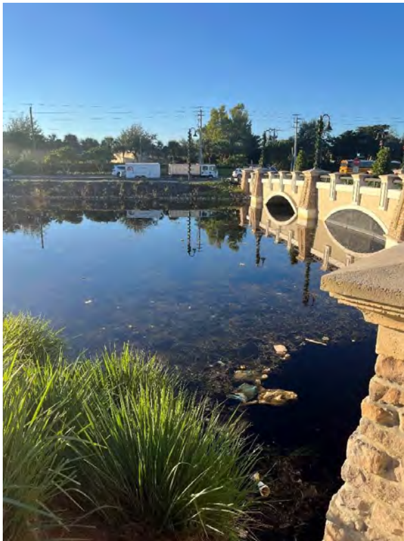
(5) Trash & Debris in canal removed
