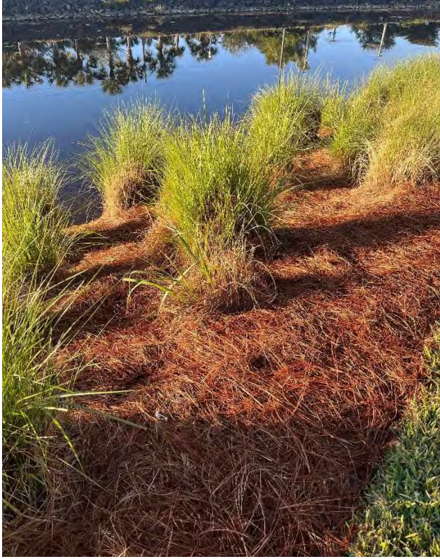
(3) New Pine Straw placed along flowway banks
